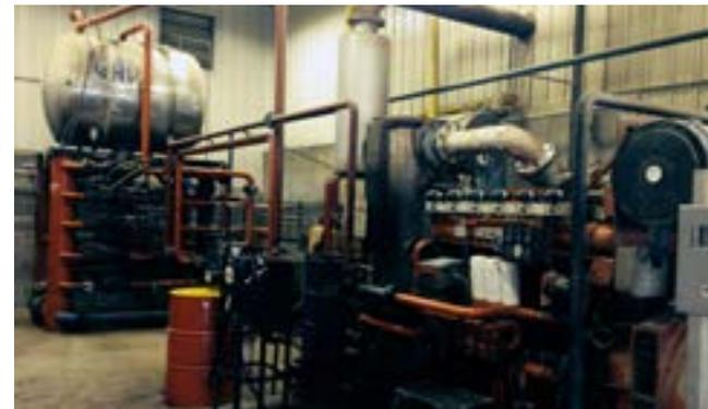
*The AD unit's electric generator is powered by methane produced with liquid dairy manure.*
