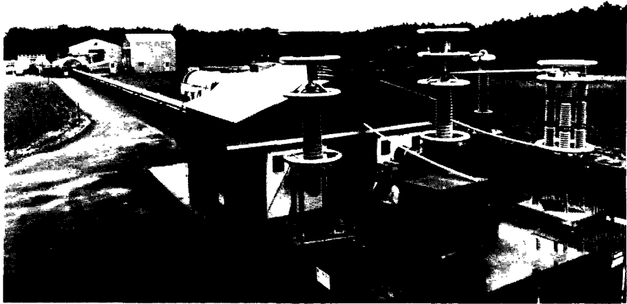
Figure 19.3. Photo of superconducting transmission line at Brookhaven National Laboratory.
