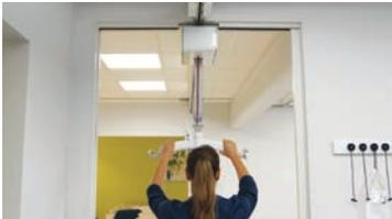
After checking that the Safety lock has engaged, position yourself right behind or in front of the hoist. It is now safe to manoeuvre the hoist through the Combi-lock, and on to the fixed or traverse rail.
