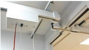
When the hoist has passed through the Combi-lock it is safe to move the traverse rail.
