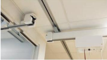
Position the traverse rail so it is aligned with the Combi-lock rail.
