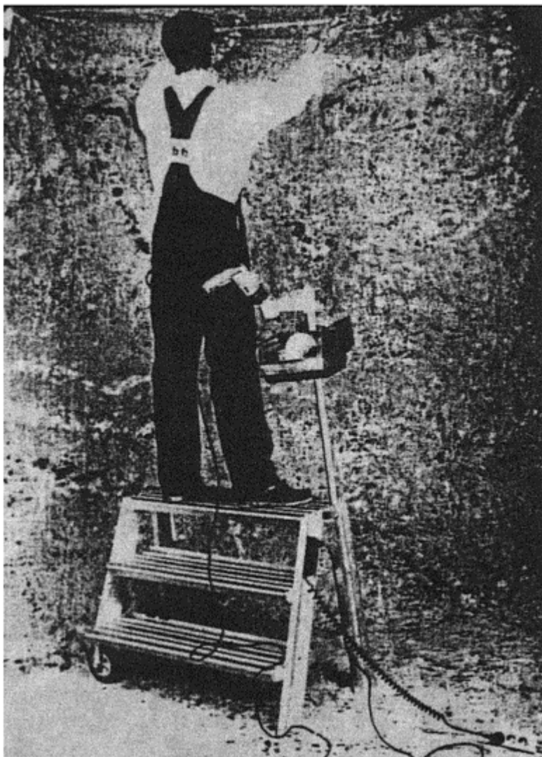
Figure 6. The new working-trestle
