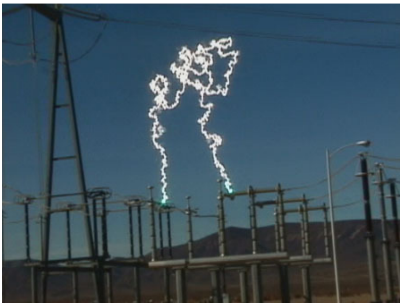
Figure 8: Photograph of a 500,000 Volt switching at Eldorado Substation in Boulder City, Nevada. Substation owned by Southern California Edison. 6
