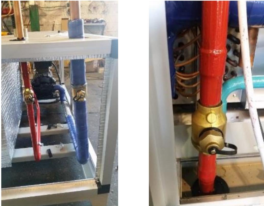
Figure 4-3. Tube stop valves
