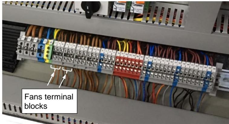
**Figure 4-6. Fan connections**
