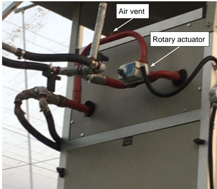
**Figure 4-9. Unit with heating/cooling**
