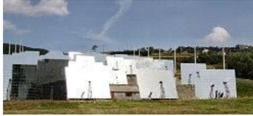
Fig: The array of mirrors is controlled by a computer and turn with the sun.
