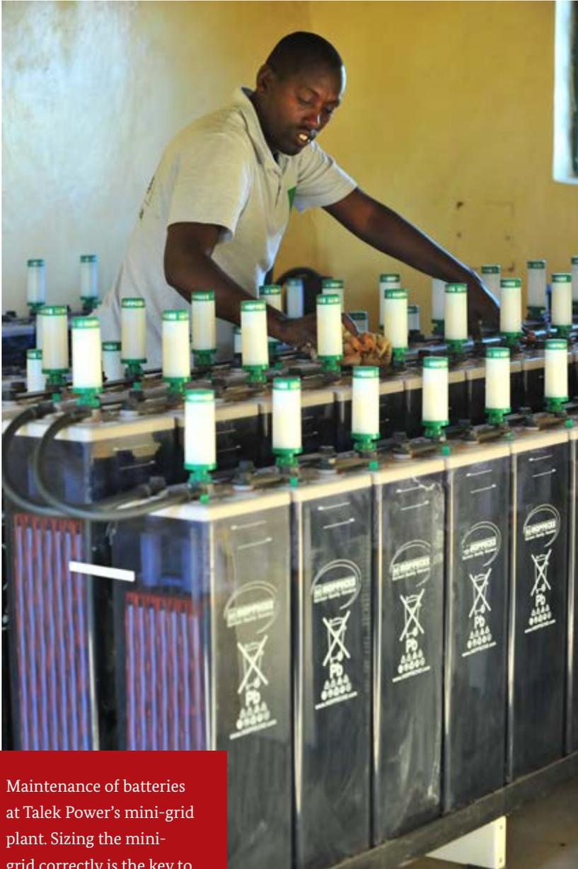
Maintenance of batteries at Talek Power's mini-grid plant. Sizing the mini-grid correctly is the key to successful performance.
