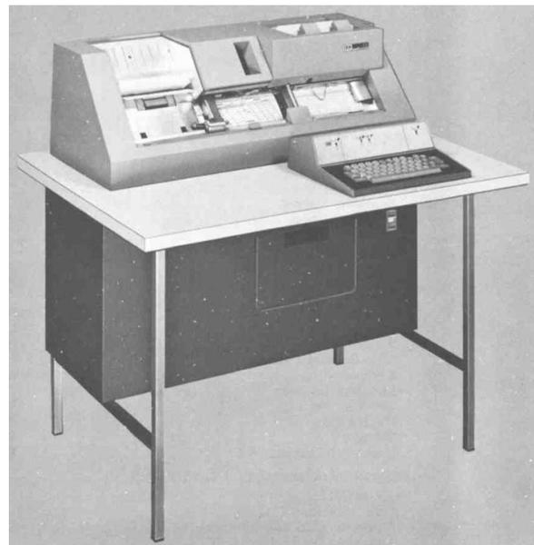
**Figure 4. IBM 029 Keypunch Machine**
