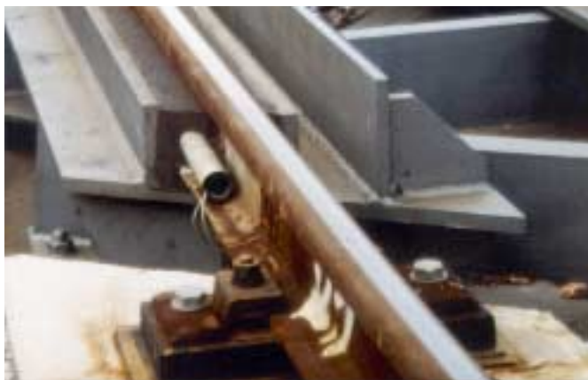
Figure 15.19: Traditional embedded rail concept on steel bridge
