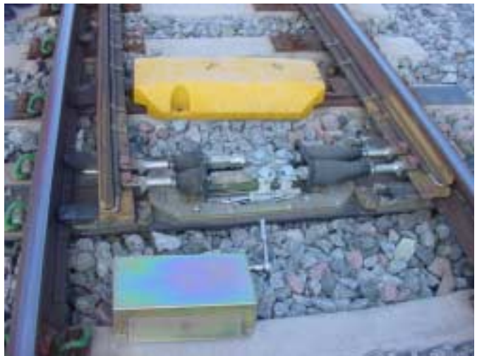
Figure 11.7: Modern electrical point machine
