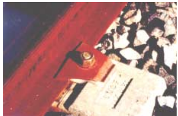
Figure 8.26: Nabla fastening system
