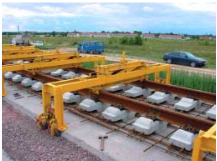
Figure 9.16: Alignment portals in the Leipzig-Gröbers project
