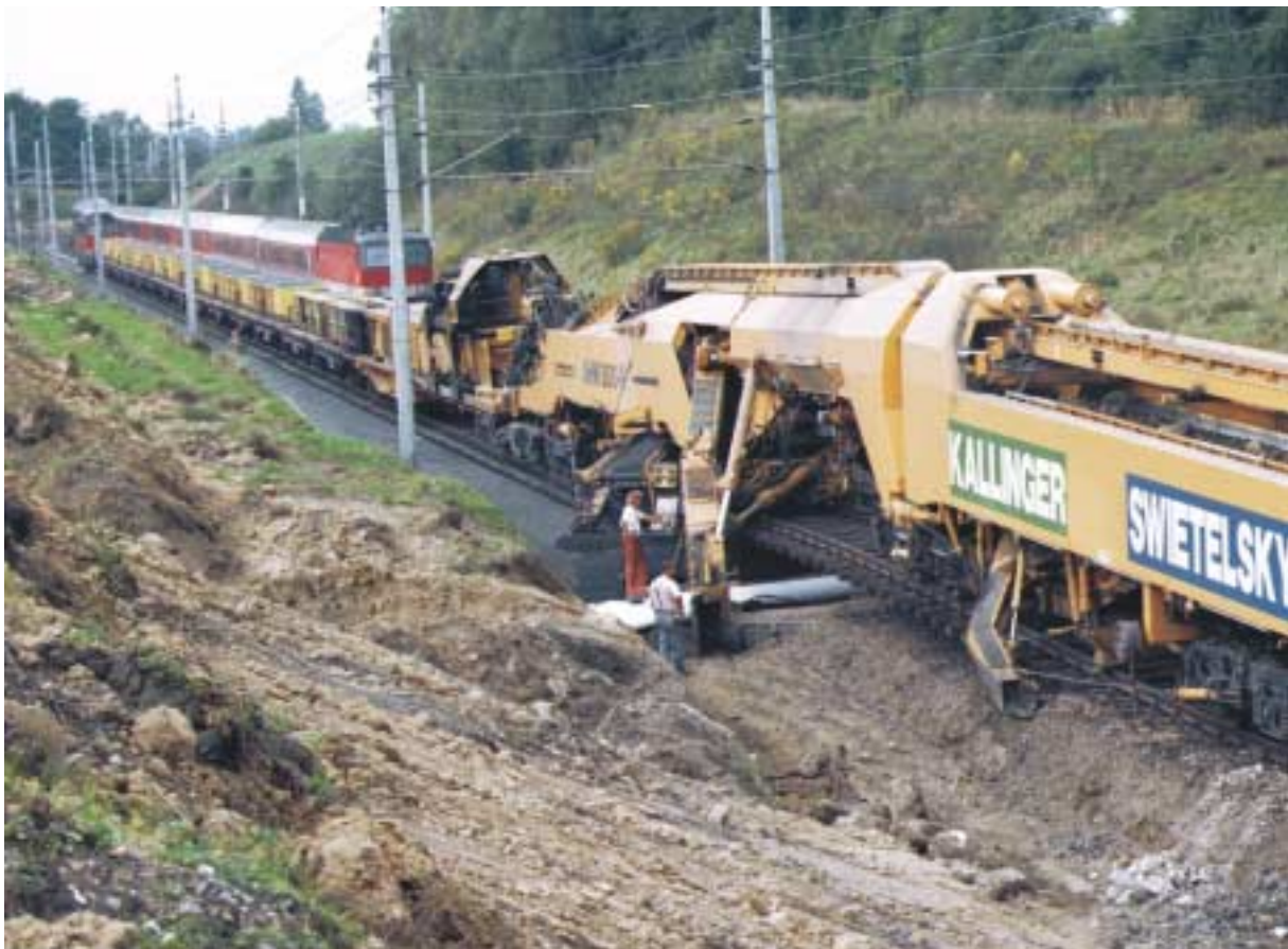
Figure 12.61: Formation rehabilitation machine AHM 800 R
