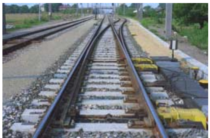
Figure 11.2: Picture of right-hand turnout
