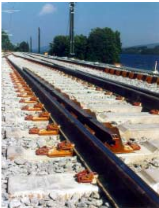
Figure 9.1: Ballasted track ...
