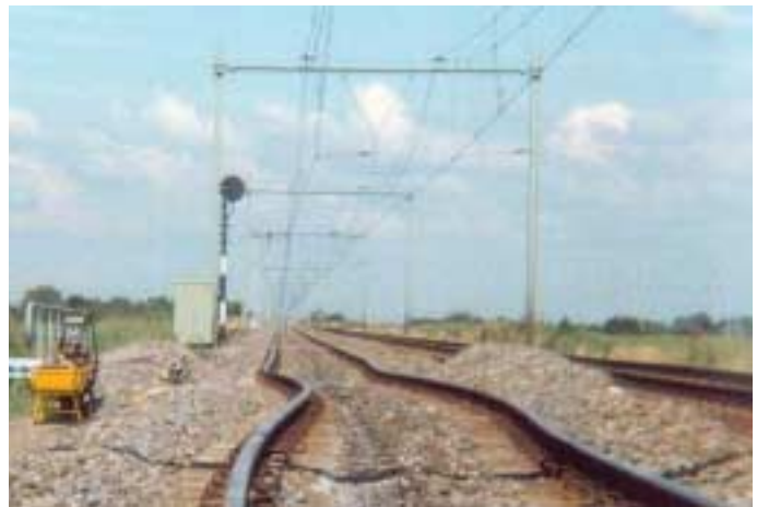
Figure 7.1: Example of track buckling
