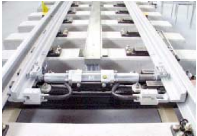
Figure 11.6: Switch with integrated hydraulic setting and locking system
