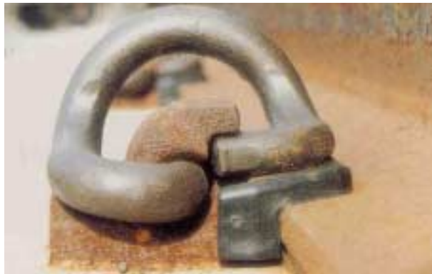
Figure 8.23: Pandrol fastening system
