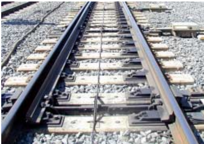
Figure 11.4: Switch blade and stock rail
