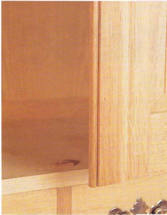
**ABOVE:** Bead to front of closing rebate, note door-stop and bolt slot
