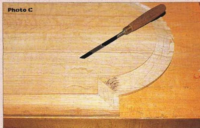
With its point in the radius's centre mark, set a trammel to the arch top mark, and draw the radius.
