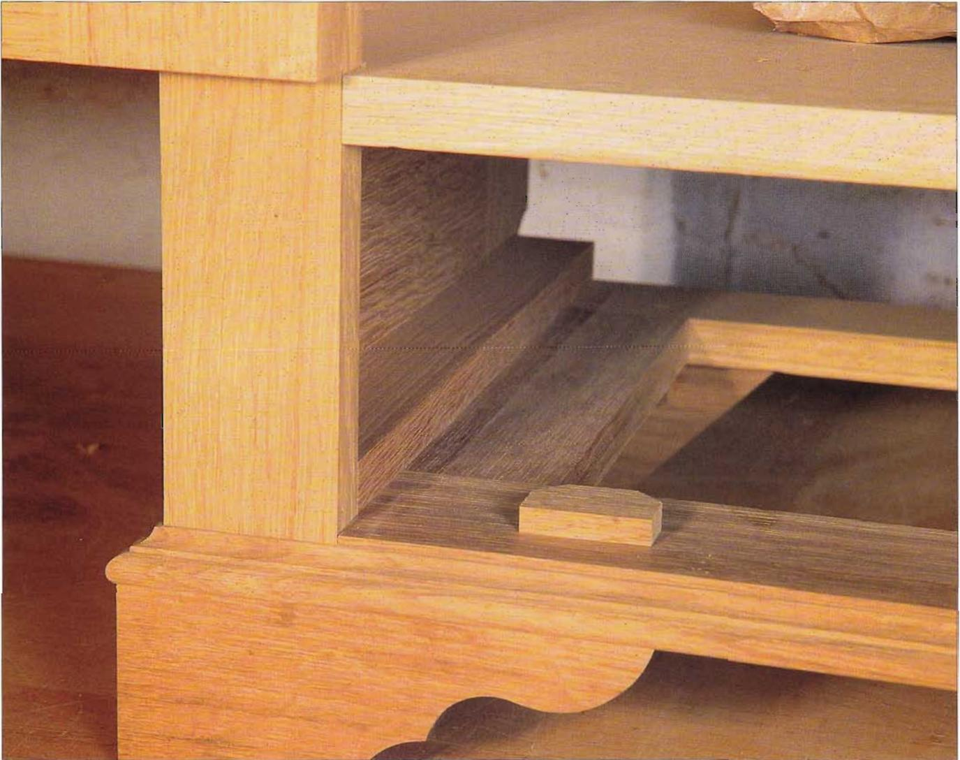
With a chest of this kind thin, fine drawer sides look wrong and are not called for, so they are finished thick enough to be grooved for the bottoms.
