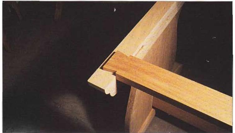
**RIGHT:** Top rails are dovetailed into the bearers – cut the tails first, then mark them onto the bearers
