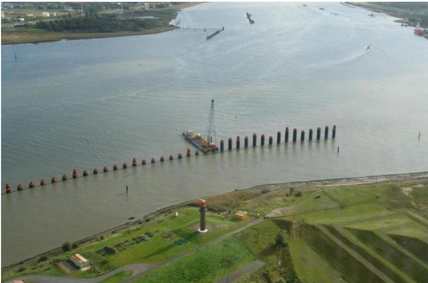
Figure 18: Construction of current deflecting wall at Deurganckdok (<http://www.hye.be/nl/news/show/one/9/>)
