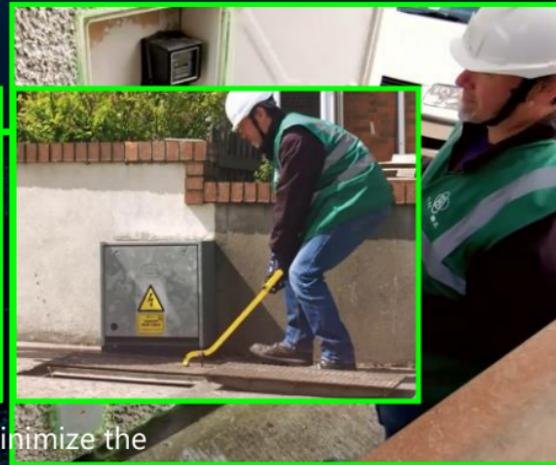
Home passed feeder cable can lay along existing ducts, to minimize the excavation
