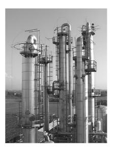
Crude oil is separated into fractions by fractional distillation. The fractions at the top of the fractionating column have lower boiling points than the fractions at the bottom. The heavy bottom fractions are often cracked into lighter, more useful products. All of the fractions are processed further in other refining units.
