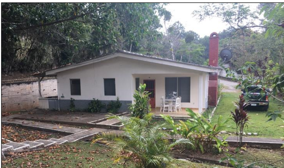
Figure 18.14 – Typical mine camp accomodation
