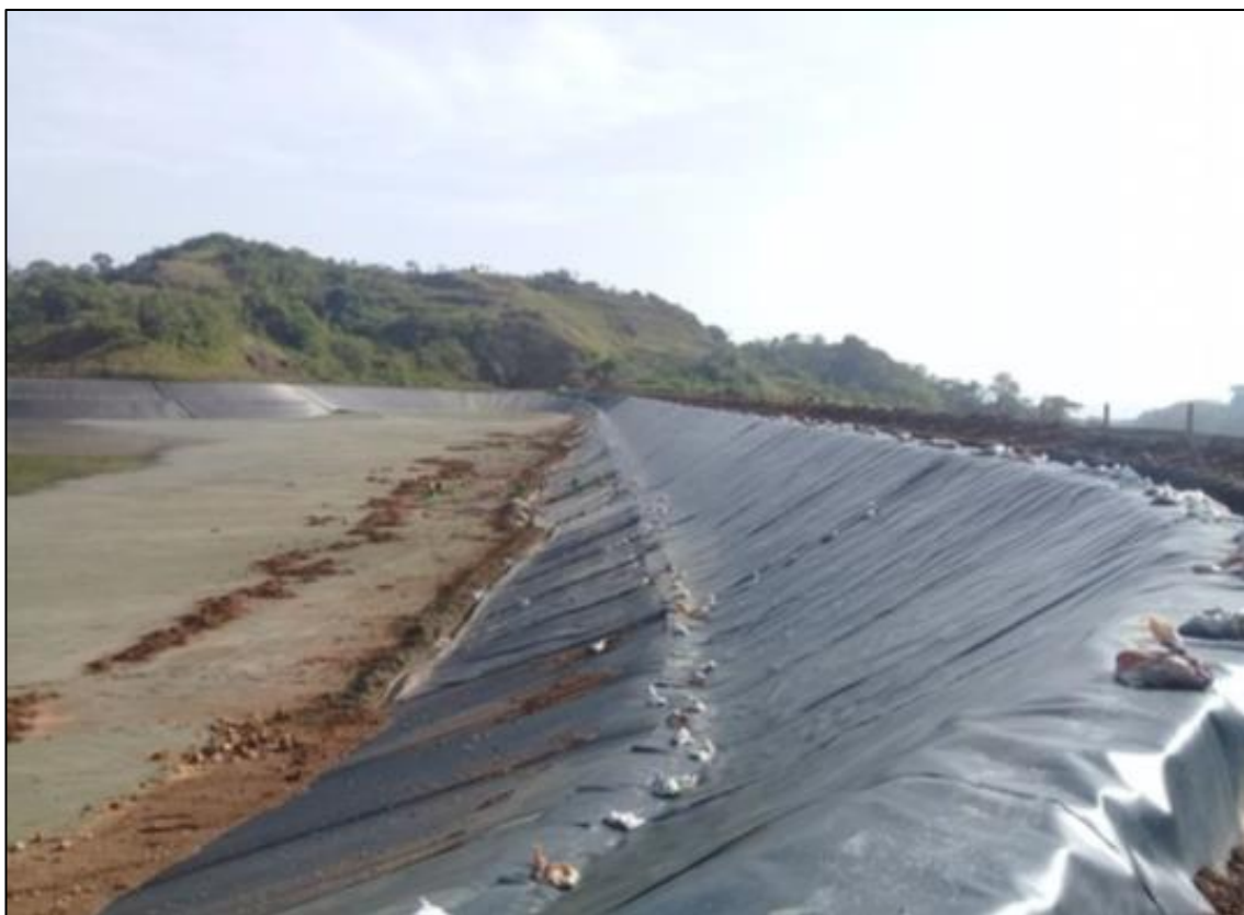
Figure 17.18 – La Soledad Dam Raising and Lining
