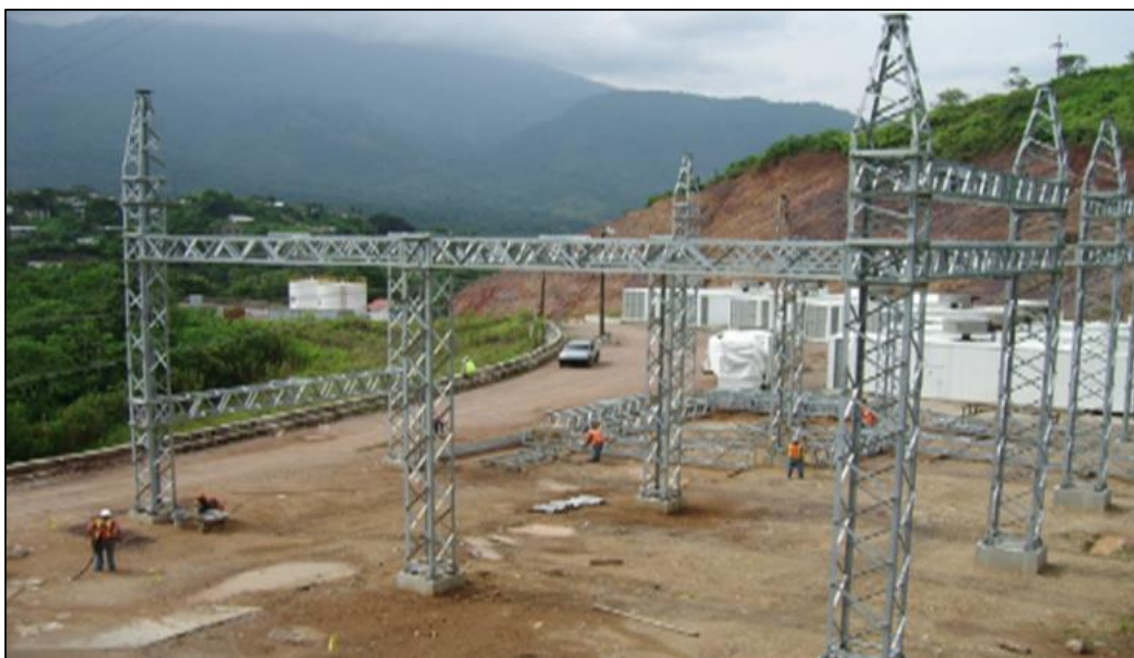
Figure 18.7 – 69 kV substation under constructions
