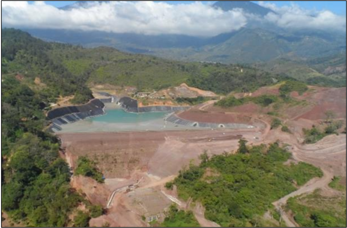
Figure 17.17 – La Soledad TSF (looking west)
