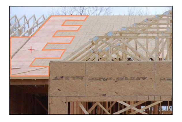
**RATIONALE:** In a group of townhouses, each townhouse must be considered a separate building from its neighbors. According to the *International Residential Code*, in order to provide the appropriate separation, using fire-retardant treated wood, along with a class C roof covering, is an acceptable alternative to using a parapet.
