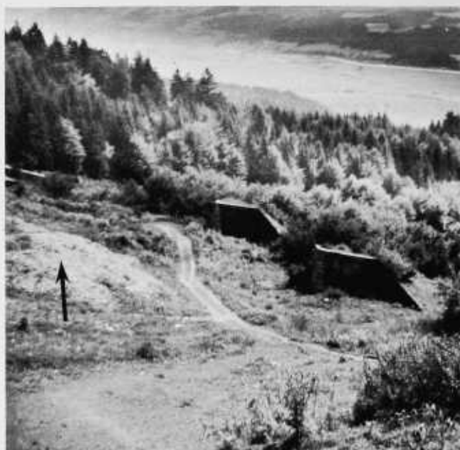
FIGURE 58.—Arzler Alm and the original system of avalanche breakers. Arrow indicated the mound of waste material which was the model for present-day design. Note natural reforestation behind the breakers.
