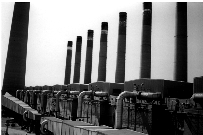
FIGURE 23.3 Large reverse air baghouse.
