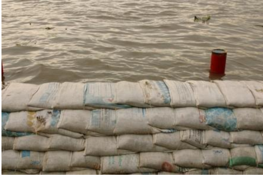
Using sand bags to prevent flooding
