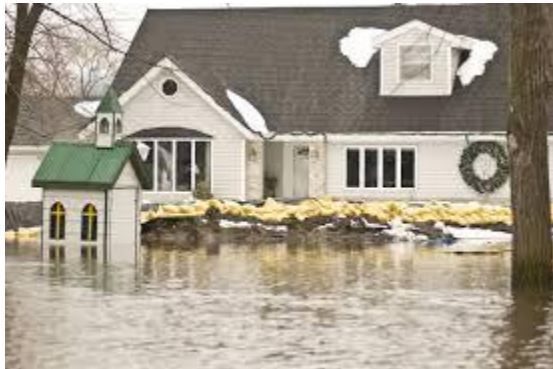
Using sand bags to prevent flooding
