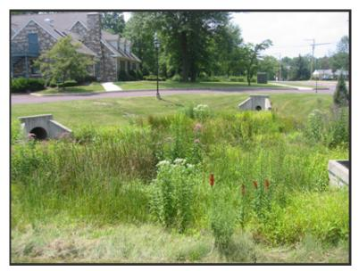
Figure 15: Stormwater wetland.
