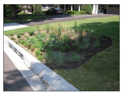
Figure 16: Bioretention cell inlet.
