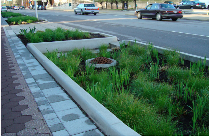
The rain garden collects and filters stormwater runoff reducing the burden on stormwater infrastructure systems.
