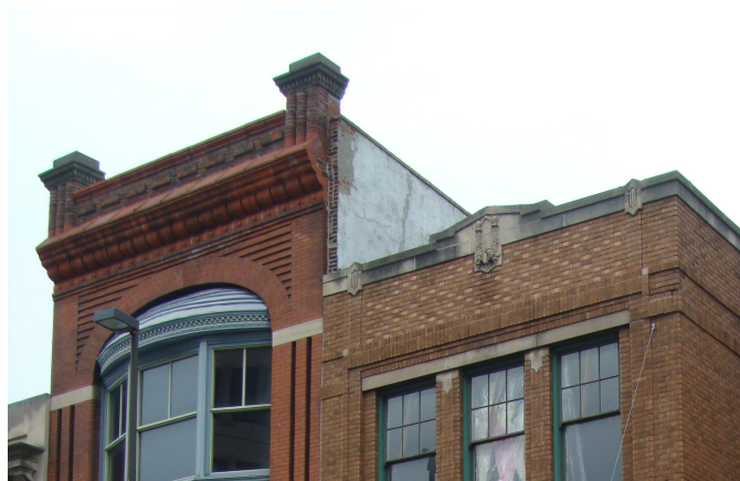
Cornices and parapet walls can be used to provide a visual termination at the top of a building.
