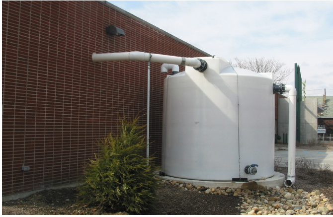
Rainwater harvesting cisterns, like the one shown above, can collect rainwater from the roof to use for landscape watering or other non-potable water needs.
