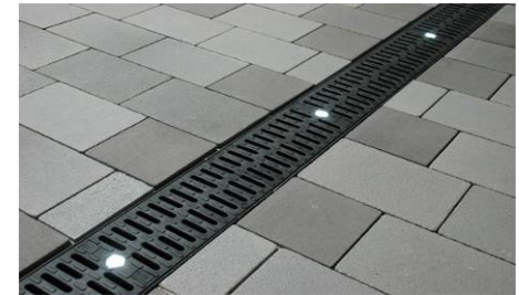
Figure 10 Closed Drainage System
