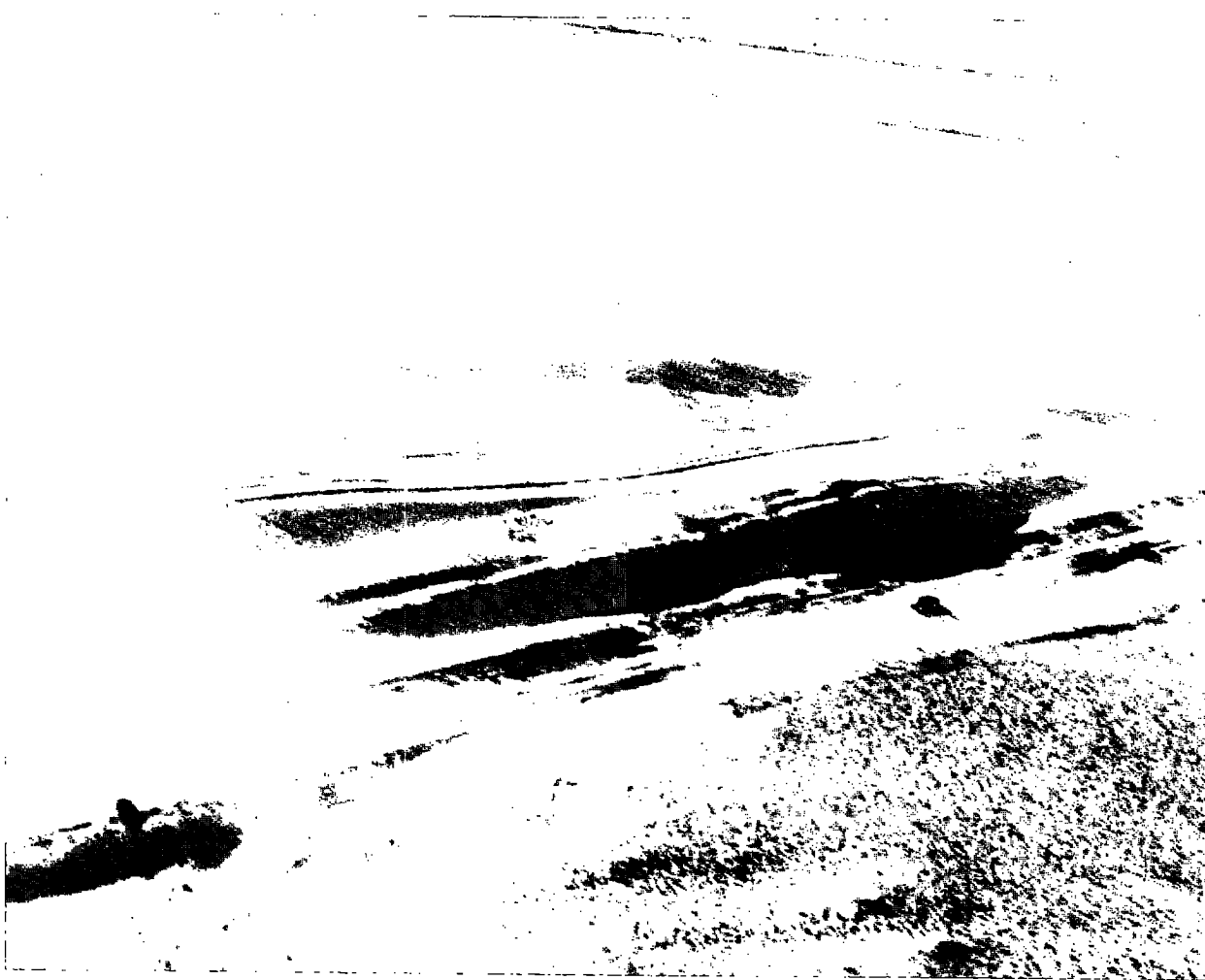
Figure 2.8. Very little blowing snow is seen escaping the two 3.8-m (12.4-ft) fences at Mile 263.0, Wyoming I-80 (Tabler 1973a). At the time of this photo, the lead fence was about 60% full. Photo by Robert L. Jairell.
