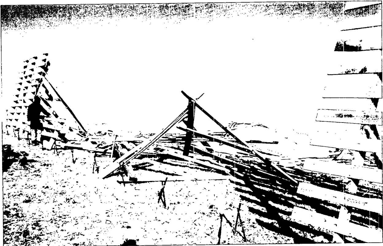
Figure 5.10. Crossed and wired rebar should not be used to anchor Wyoming fences.
