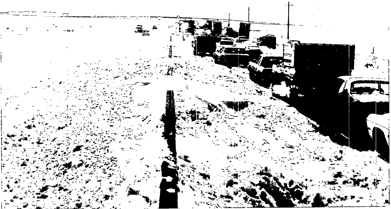
Figure 7.28. Concrete barrier caused a snowdrift that blocked Interstate Highway 25 in Colorado, during the Christmas blizzard of 1982.
