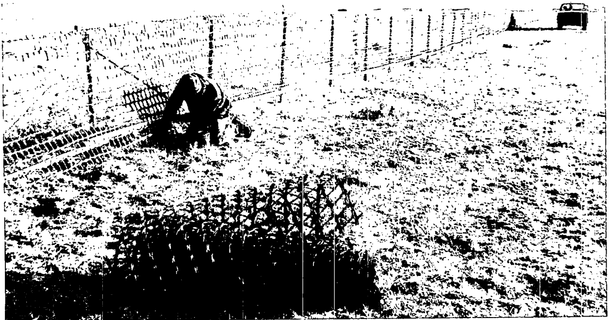
Figure 5.19. Extruded high-density polyethylene “L-300 Sand and Snow Fence” manufactured by DuPont Canada Inc.
