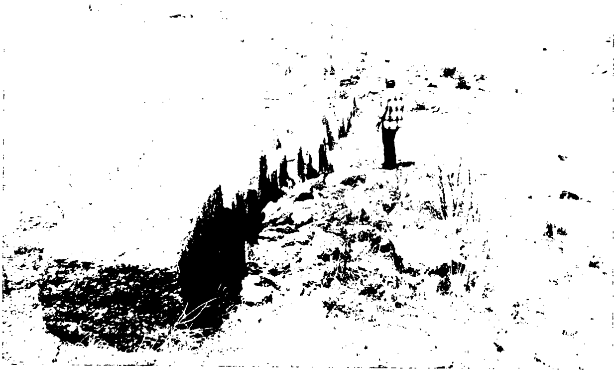
Figure 2.1. Rock snow fences protecting railroad cuts in southeast Wyoming were probably built in 1868 (Tabler 1986).
