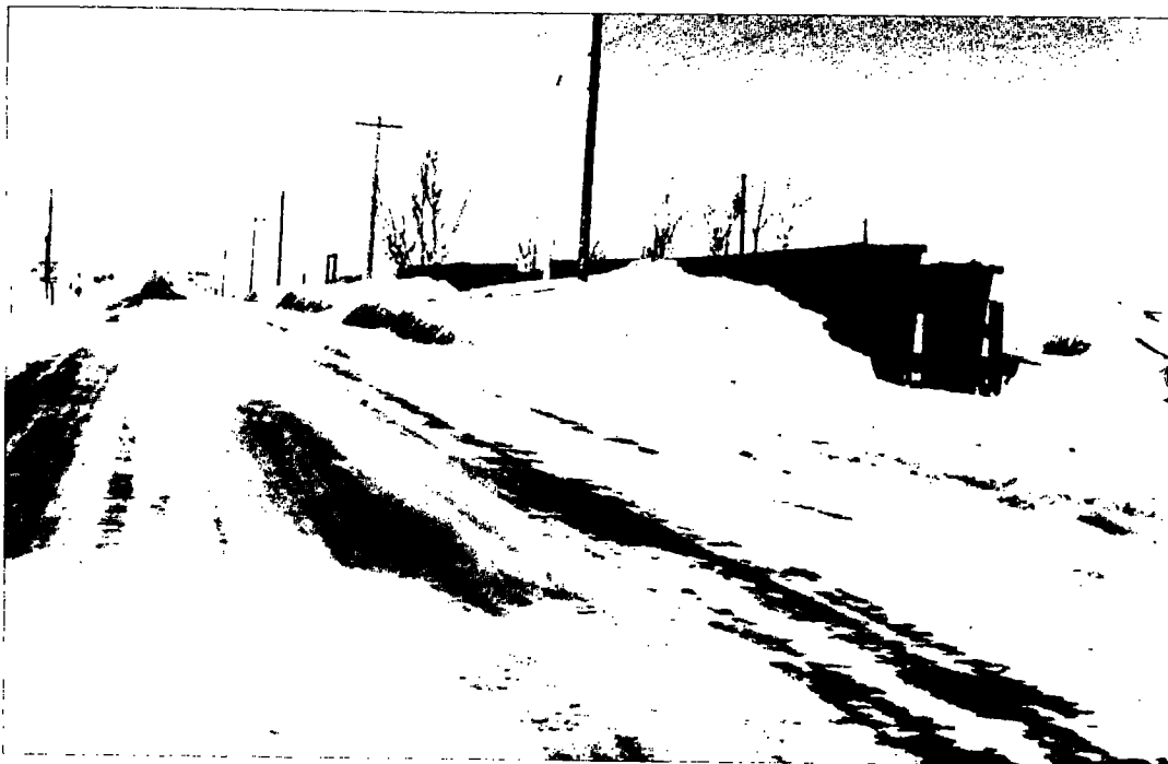
Figure 4.1. A board fence, 2.4-m (8 ft) tall, that caused a drift on the road. Wind was from left. Structures and vegetation on the downwind side of the road are sometimes overlooked during summertime field reviews.
