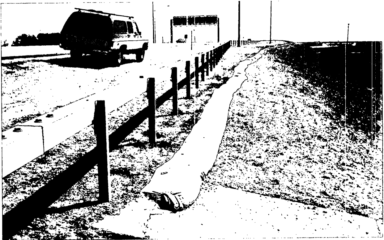
Figure 7.30. A temporary curb comprised of a sand-filled canvas or plastic sleeve, should be used in preference to permanent curbs under rail.
