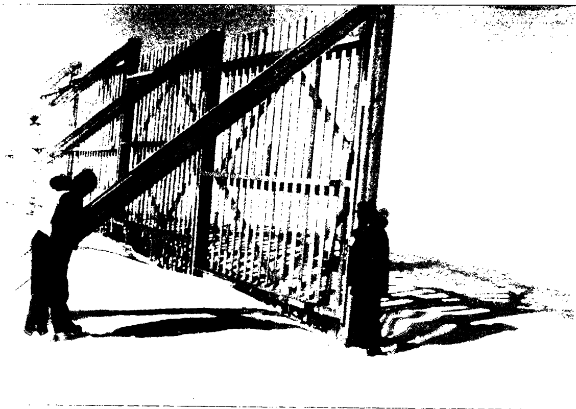
Figure 5.17. Vertical slats supported by horizontal stringers between vertical supports were used for this 4.6-m-tall (15 ft) fence at Wainwright, Alaska. Photo by George Clagett, U.S. Soil Conservation Service.
