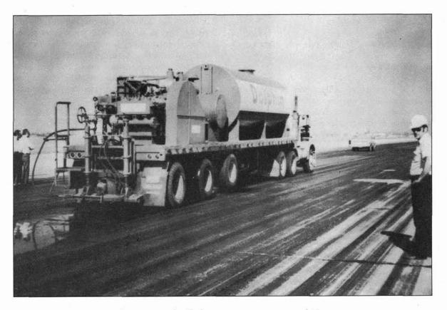
Figure 8-1. Oscillating high-pressure water vehicle
