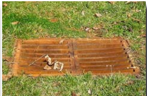
Drop Inlet in Yard
