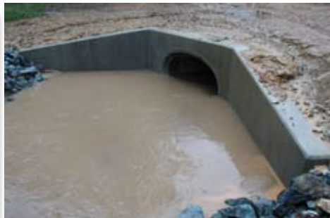
Head Wall - Concrete
