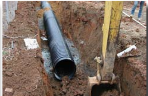
High Density Polyethylene Pipe (HDPE) Installation
