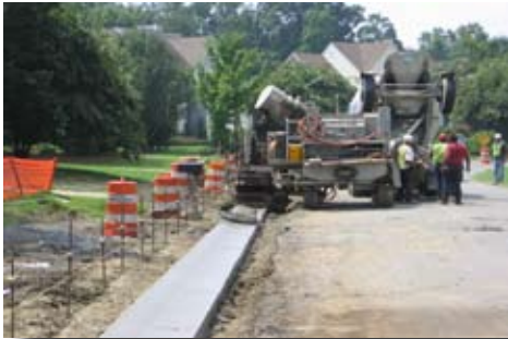
Curb-Gutter Installation
