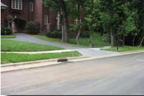
2' 6" Standard Curb and Gutter
