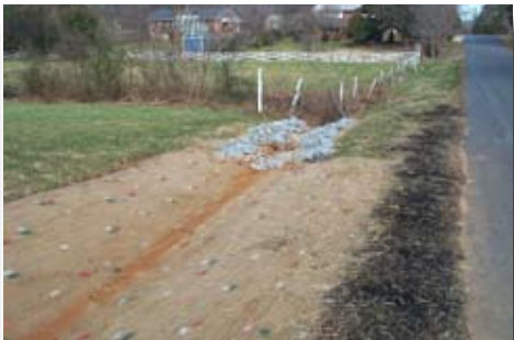
Temporary Erosion Control Matting
