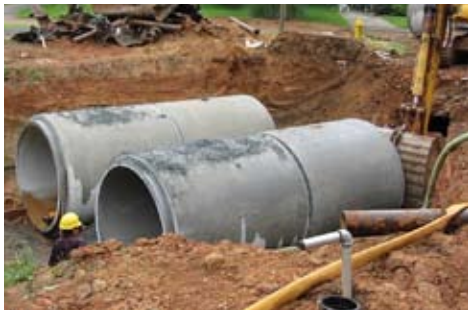
Reinforced Concrete Pipe (RCP) Installation
