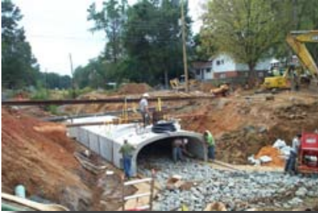
Bottomless Culvert - Arch
