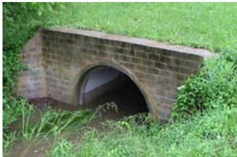
End Wall With Wing Walls
