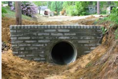
Head Wall - Concrete Block
