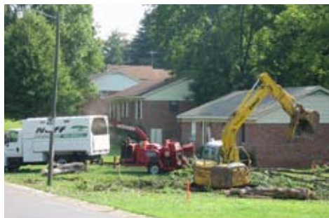
Tree Removal - Chipping
