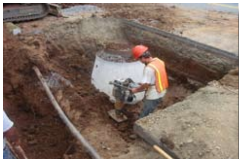
Backfill Tamping with Jumping Jack
