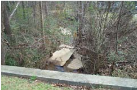
Concrete in Stream
