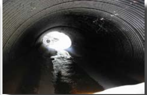
Corrugated Metal Pipe (CMP)
