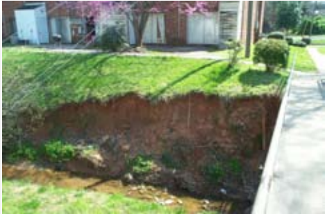
Channel Erosion
