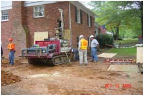
Micropile Drill Rig
