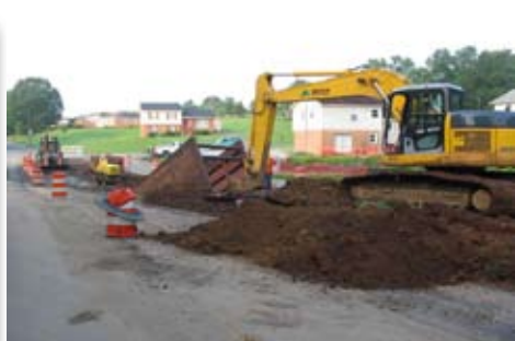
Trenching in the Street
