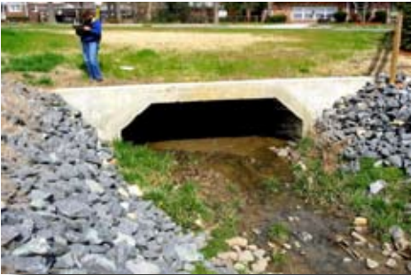
Bottomless Culvert - Three Sided
