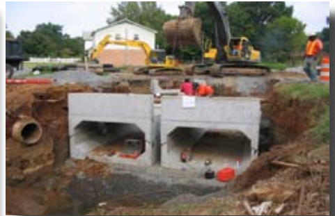
Double Reinforced Concrete Box Culvert (RCBC)
