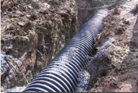
High Density Polyethylene Pipe (HDPE)
