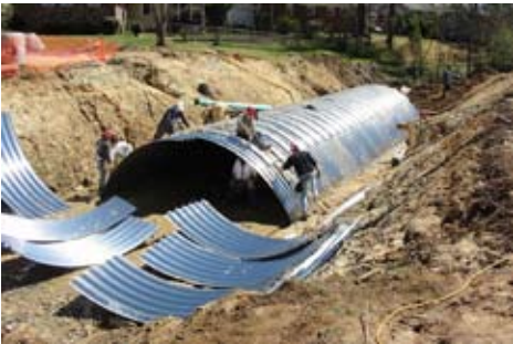
Corrugated Aluminum Pipe Arch (CAPA)
