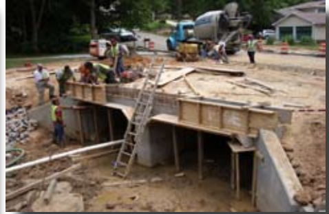
Head Wall Under Construction
