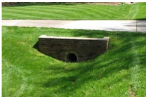
Head Wall - Brick
