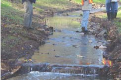
Grade Control Structure
