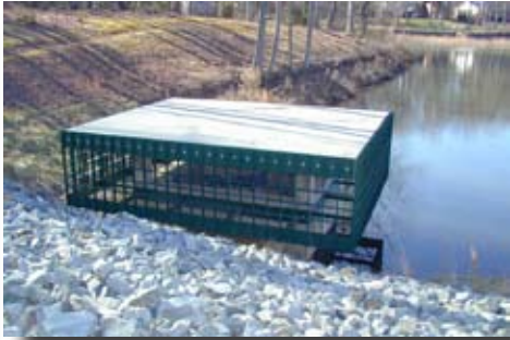
Pond Outlet Structure with Trash Rack
