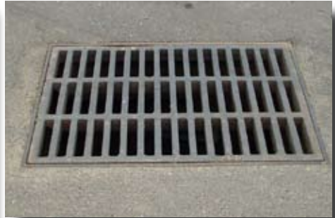
Drop Inlet in Pavement
