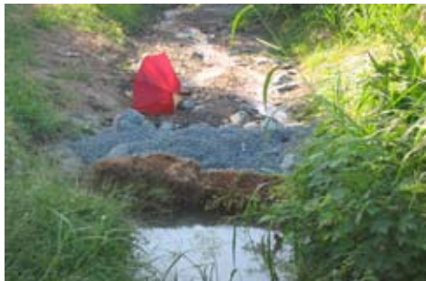
Temporary Rock Check Dam
