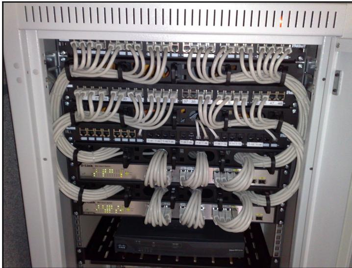
Figure 6.14: Front of the patch panel
