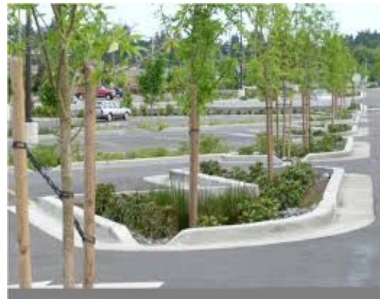
Biofiltration with trees in Island
