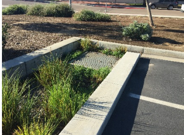
An overflow outlet conveys runoff that exceeds the biofiltration area capacity
