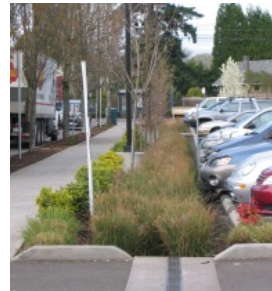
Bioswale adjacent to parking and sidewalk
