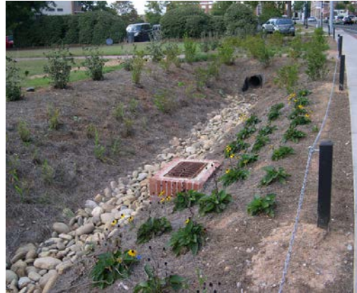
Swale outside of sidewalk and road
