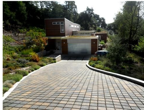
Permeable pavement driveway
