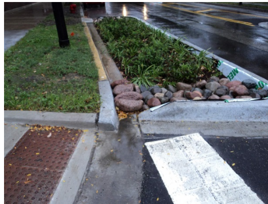
Bulb-out at intersection
