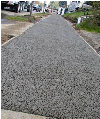
Pervious concrete sidewalk
