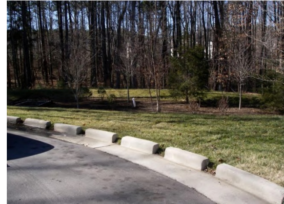
Curb cuts with filter strip
