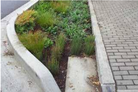
Permeable pavement sidewalk with biofiltration
