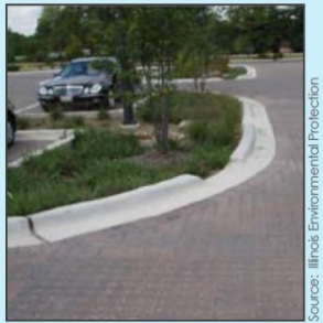
A curb inlet directs runoff into a biofiltration planter
