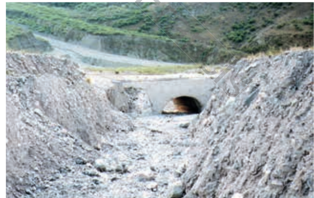
Photo D Silting of riverbed to above road level, requiring excavation to an artificial channel, northwest Argentina.
