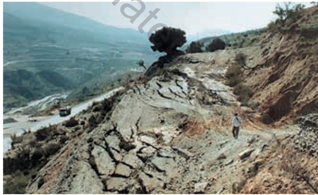
Photo E Damage to motorways caused by landslides, southern Spain.
