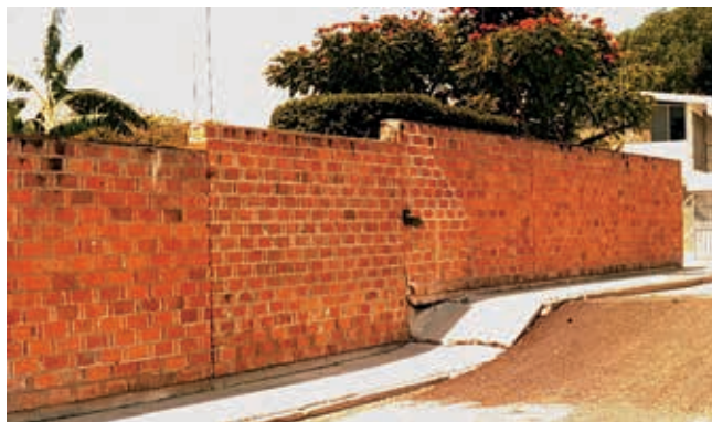
Photo F Subsidence along active faults caused by water extraction from wells, Celaya, Mexico.
