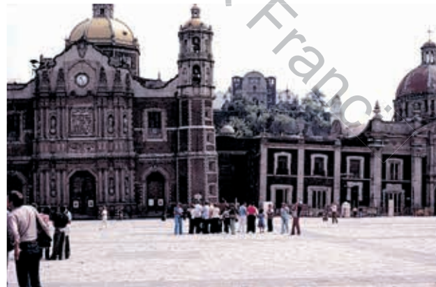
Photo D Settlement of the basilica N a S a de Guadalupe, Mexico City, built on soft lacustrine soils affected by subsidence.
