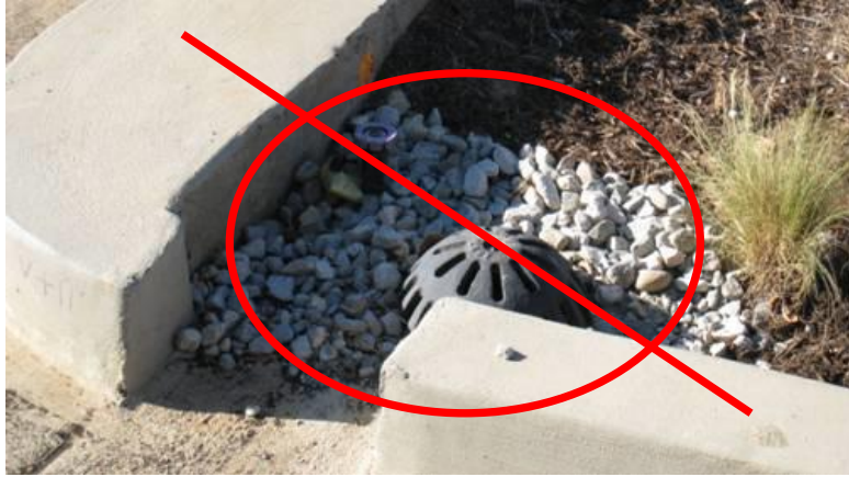
Figure 6: Incorrect Placement of an Overflow Inlet
