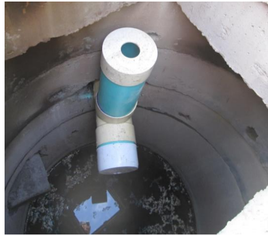
Figure 1. Example Outlet Control Structure
