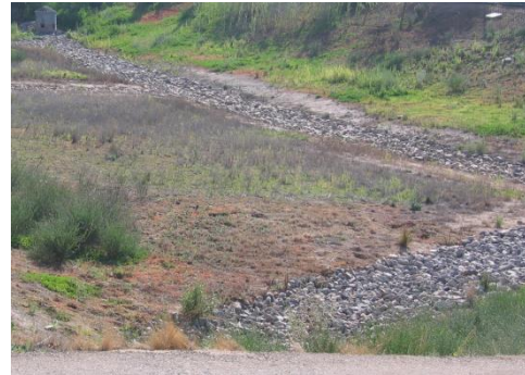
Figure 3: Gravel filled low-flow trench
