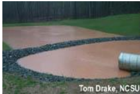
Figure 2: Forebay filled with storm water
