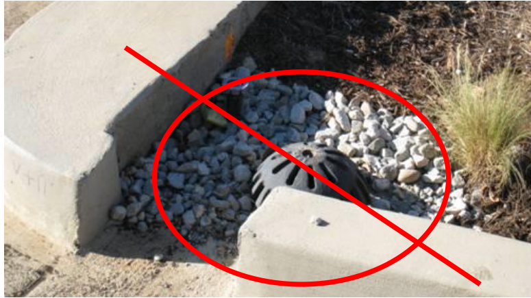
Figure 5: Incorrect Placement of an Overflow Inlet
