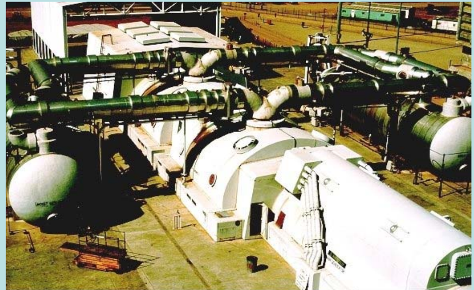
Overview of a steam turbine and main generator for a nuclear steam power station. (Courtesy of Carolina Power and Light Company)
