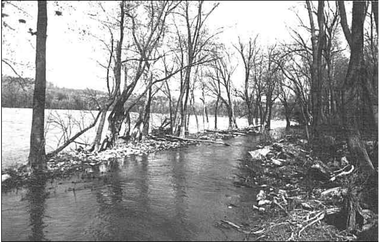
Figure 20. Peacher's Mill millrace. The millrace is currently clogged with dead wood and other flood debris. (Photo by Rob Brzostowski)
