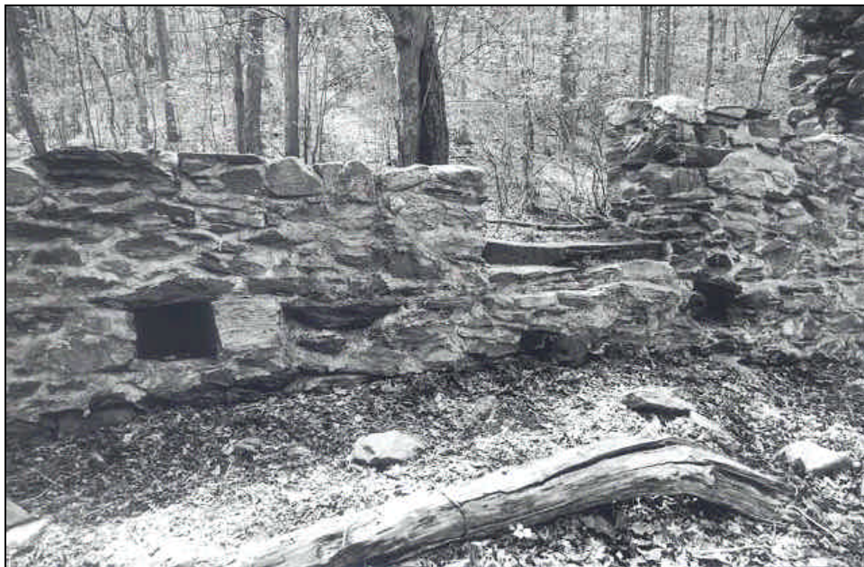
Figure 22. Timbers were inserted into these square joist pockets to support the millstones on the first floor. (Photo by Rob Brzostowski)
