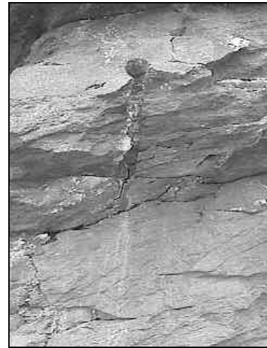
Figure 16. Quarrying and black powder blasting was necessary to open parts of River Road. Drill marks such as this are evidence of the techniques used. (NPS photo by Andrew S. Lee)
