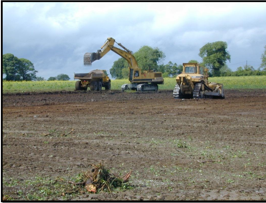
Plate 2 – Soil stripping by backhoe and dumptruck
