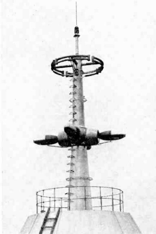
FIG. 169.—Radiator system designed by Lindenblad for station W2XBS, the National Broadcasting Company's transmitter atop the Empire State Building in New York City. The top structure is the folded dipole used for sound transmission, the lower the constant-impedance turnstile structure for the picture signal.
