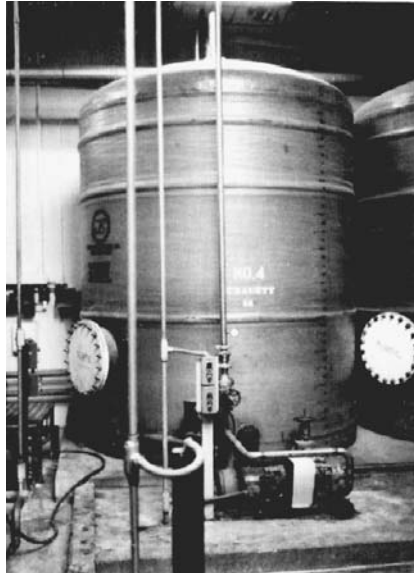
FIGURE 6.6.2i 5000-gal tank made by the filament-winding process. (Courtesy Justin Enterprises and Johns-Manville Corp.)
