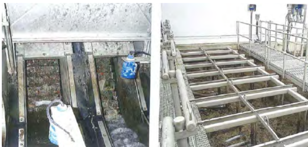
Figure 8.9 process stages at the Markranstadt wastewater treatment plant. Left: step screen, right: nitrification and de-nitrification tanks
