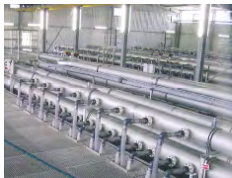
Figure 8.5 membrane installation at the WWTP Nordkanal
