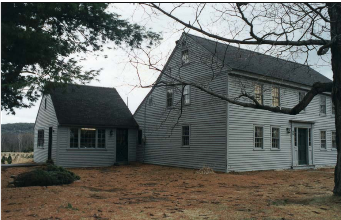
A lean-to (or saltbox) roofline, massive central chimney (since removed from this house), center entrances, and facades with regularly spacing of door and window openings were common features in 18th century farmhouses.
