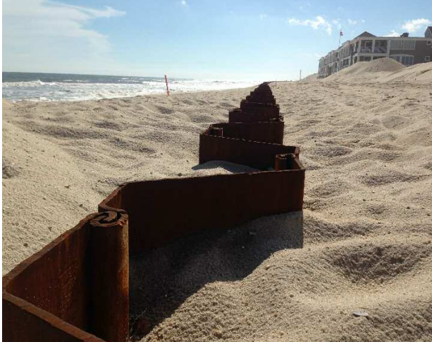
Figure 14. Sheet pile dune core (picture taken shortly after installation, before it is capped and buried by the dune), in Brick Township, New Jersey.
