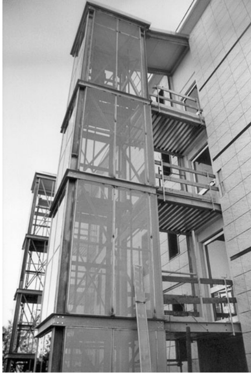
FIGURE 15.4 The renovation project of a deteriorated neighborhood of the 1960s in the small city of Pinerolo, northern Italy, provided for better energy efficiency and accessibility in the four-story buildings with a large number of older adults. Further, a stair lift was installed near the entrance to allow accessibility to and usability of the first-floor apartments.
