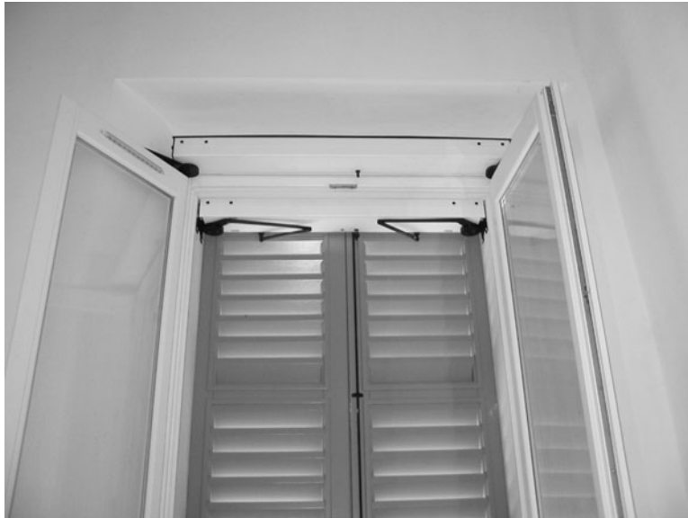
FIGURE 15.3 The renovation project in Bagnacavallo included the removal of old windows, which were replaced by motorized windows and shutters, to be easily operated by the residents.
