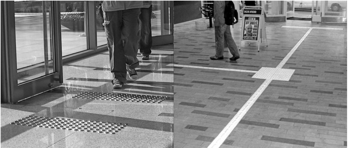
FIGURE 42.5 Two types of markings. Steel knobs as found in front of the main entrance door to the Severance Hospital in Seoul (left) are fairly common. The Danish solution (right) in Kalundborg Central Station, made from white steel tiles, uses both tactile and contrast color. [Photos: Jon Christophersen (left); Dansk Blindesamfund (right).]
