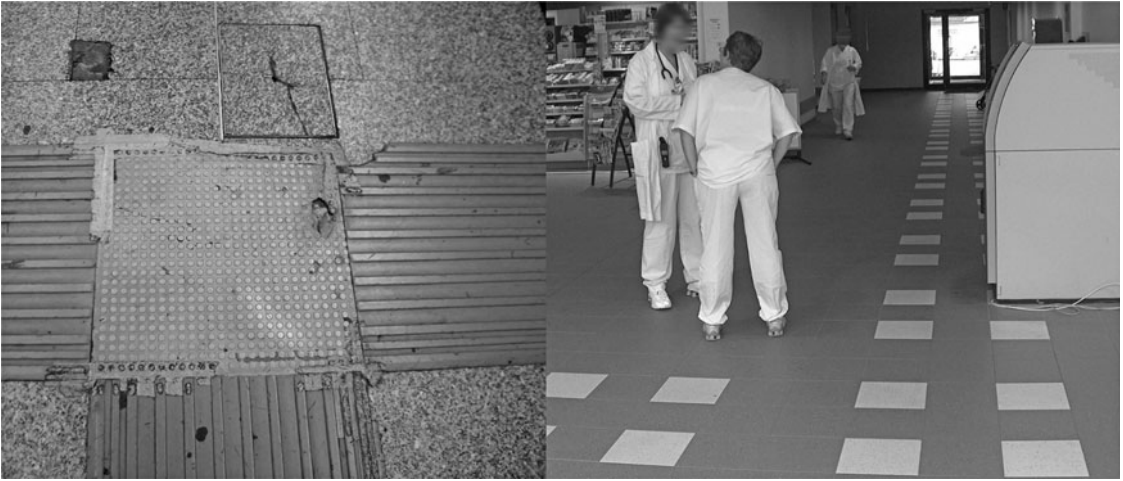
FIGURE 42.6 Guidepaths have to be properly maintained—not as in the left photograph. They must also be left unobstructed; conflicts such as in the left photo must be avoided. [Photos: Karine Denizou (left); Jon Christophersen (right).]
