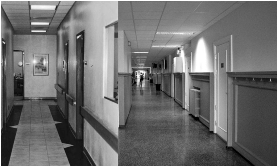
FIGURE 42.2 Left: A combination of wall and floor markings in San Diego Center for the Blind. Right: Markings on the walls of a corridor in Ullern Finishing School, Oslo, Norway. [Photos: Roberta Null (left), Karine Denizou (right).]
