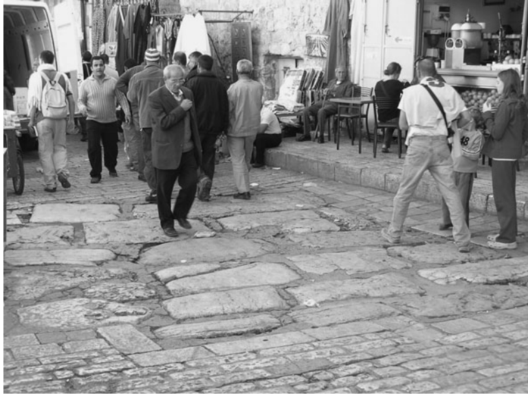
FIGURE 16.5 Via Dolorosa, with original Roman pavement in situ. A section of the Via Dolorosa is paved with original large Roman stone tiles and is combined with much smaller stone tiles of the twentieth century. Pedestrians, carts, and wagons use the pavement intensively on a daily basis.
