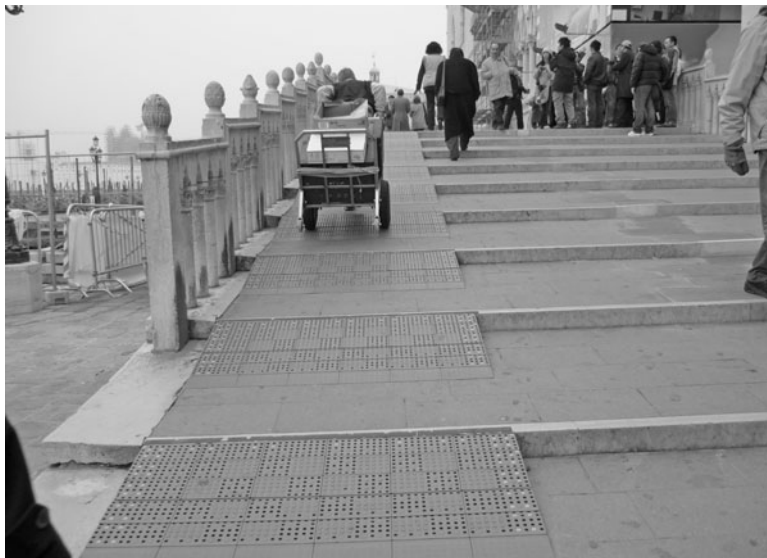
FIGURE 15.7 In recent years the municipality of Venice, Italy, has been engaged in an initiative to install mobile ramps on existing bridges.
