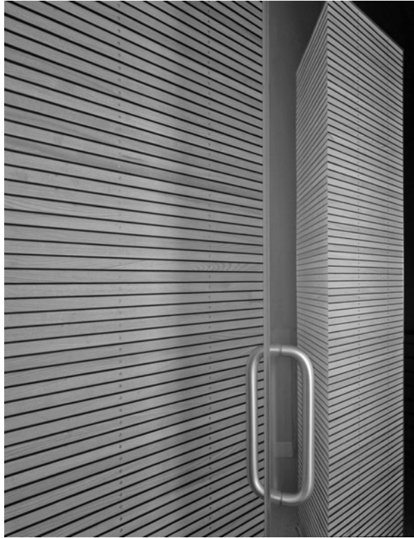
FIGURE 27.6 The bathroom wall surface in the La Marche Residence in Derby, New York, is made of protruding thin rubber strips separated by strips of ash, resulting in a wall that can be used to squeegee off water after a shower and massage the back. (Photograph © 2006 William Helm.)
