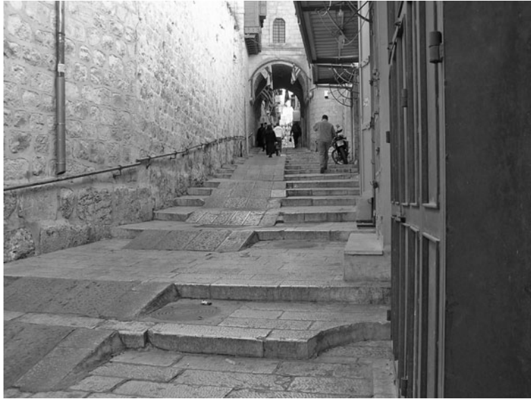
FIGURE 16.3 Semicommercial street in the Christian Quarter. A street constructed as a stairway is paved by limestone tiles, and a handrail is mounted on the left façade wall. Narrow stone ramps are anchored into the stairway for scooter and wheelchair users as well as pushers of carts and wagons.
