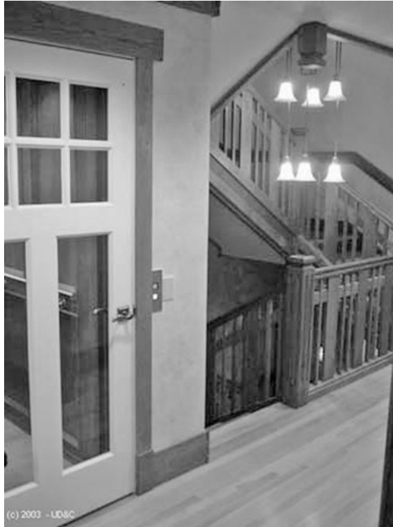
FIGURE 26.6 The cherry stairwell includes craftsman details in the handrails located on both sides. The newels and columns create a forest of grippable surfaces while the adjacent elevator with exterior windows and glass doors provides comparable access to all floors.
