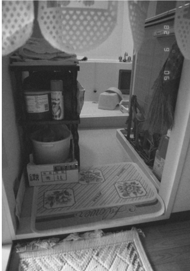
FIGURE 11.1 Level changes to enter a bathroom. There exist two level changes, one between the wooden floor and clothing area, the other between the clothing area and the wet area of the bathroom. This is a bathroom in a dwelling unit for frail seniors built around the late 1980s.
