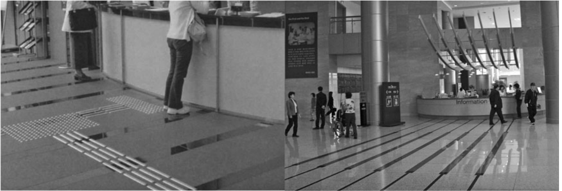
FIGURE 42.1 Guidepaths in floor surfaces. Left: Knobs attached to the flooring material. Cones signal a change of direction; tongues indicate the line of flow. Right: Dark lines indicate the direction of the flow (Severance Hospital by Ellerbe Becket, Jung Lim Architects, and Kesson International, Seoul, South Korea). [Photos: Ed Steinfeld (left), Jon Christophersen (right).]
