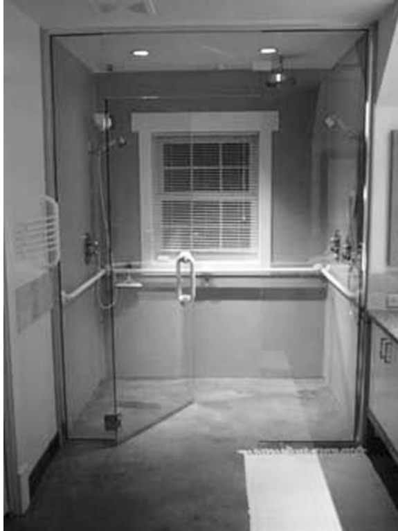
FIGURE 26.7 The curbless master shower features a stained concrete slab floor that allows a roll-in entry, a handheld shower, and horizontal white grab bars.
