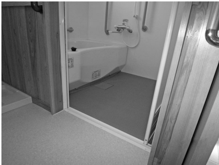
FIGURE 11.3 The water channel is almost invisible in a newer design. The water channel at the bathroom door is almost eliminated in a more recent design, which was installed in 2007 as a bathroom unit for public rental housing. In repeated experiments and practical experiences regarding water overflow, problems were solved with more sophisticated designs.
