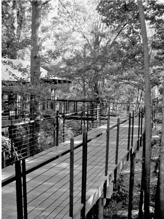
FIGURE 40.1 The entry to the tree house is a 40-ft bridge providing universal access to the tree house which stands 22 ft above the ground.
