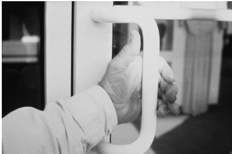
FIGURE 32.7 Open-loop door handles accommodate hands of all sizes.
