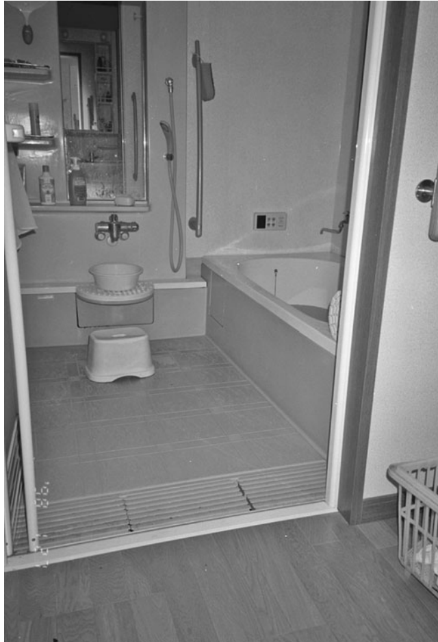
FIGURE 11.2 The level change between clothing area and wet area is eliminated in the dwelling. To facilitate this, a wide water channel exists between the two spaces. This was designed and built between 1996 and 1997 as a standard design feature.
