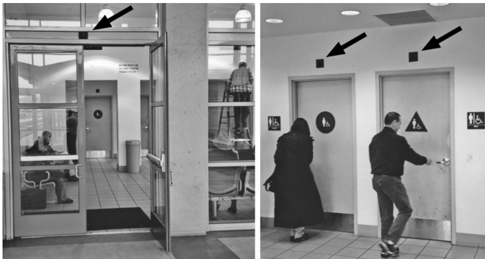
FIGURE 19.2 The CALTRANS commuter train station in downtown San Francisco is equipped with remote infrared signs or “talking signs.” They are installed above doors to key spaces such as entry doors and entries to public bathrooms.
