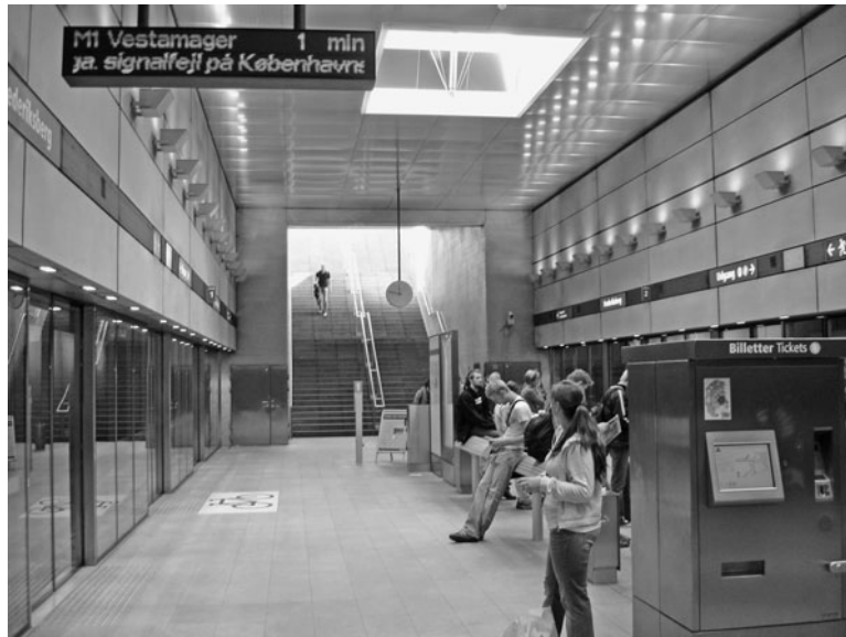
FIGURE 19.4 Safety barrier at station in Copenhagen Metro. The station is a good example of universal design features that enhance usability and safety for all, including full-height glass safety barriers with sliding doors along the platform edge, real-time arrival information on an electronic overhead sign, and well-marked route information with high-contrast fonts and directional arrows. Boarding locations are marked on the platform with tactile guide strips and is lit with natural light from a skylight above. Both seating and leaning bars are provided.
