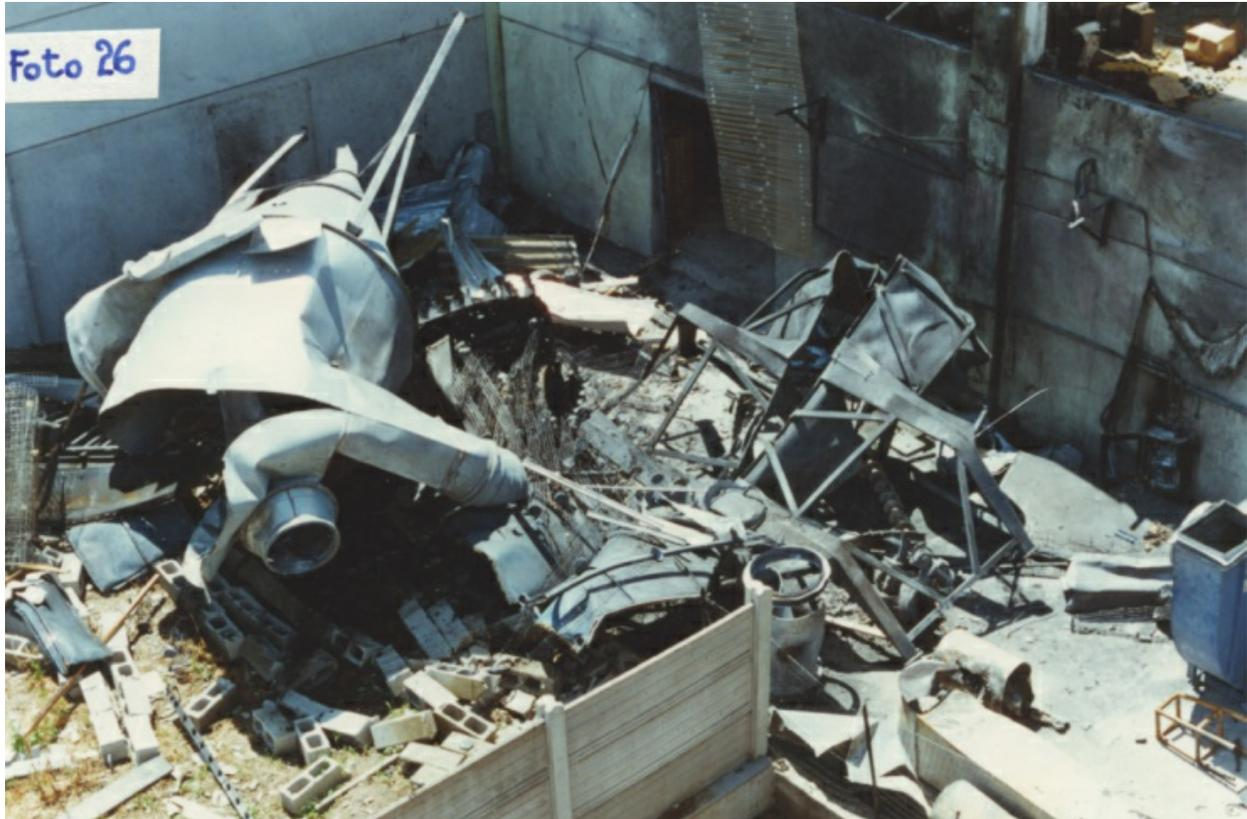
[Figure 4.27](#) State of places and damage to the abatement system.
