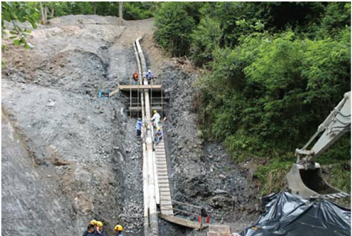
[Figure 7.9.2](#) Oil pipeline formed by two pipes with different diameter: 16” pipeline was affected by the rupture. Images show the pipeline after the excavation to sample the broken segment.
