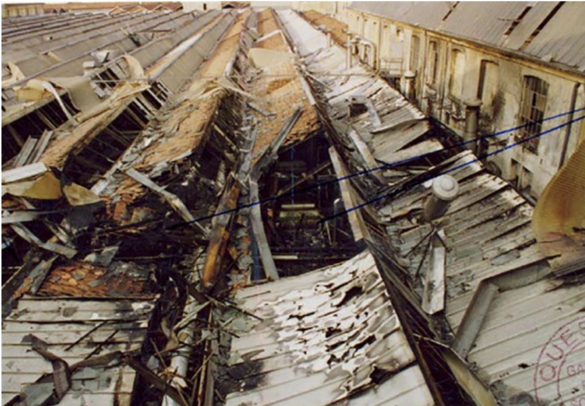
[Figure 4.20](#) Explosion of wool burrs, state of places.
