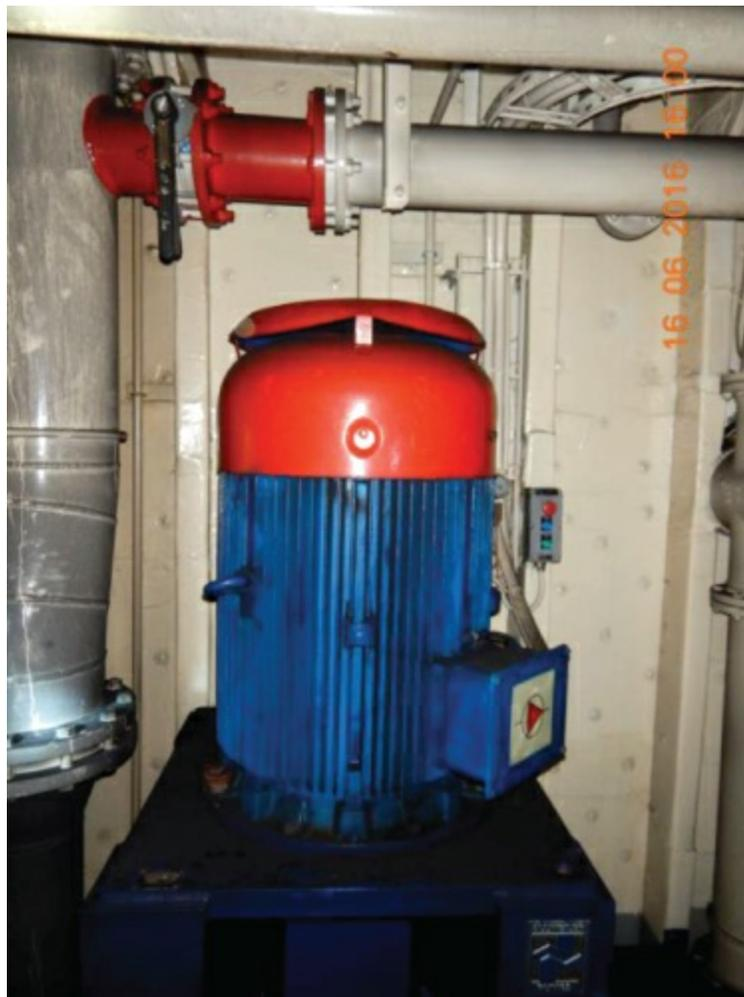
[Figure 7.2.3](#) Closed intercept valve between the emergency pump and the drencher collector.
