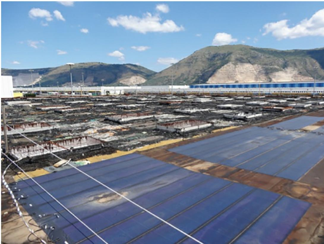
[Figure 7.10.1](#) Photo of the burned roof and the installed PV system.
