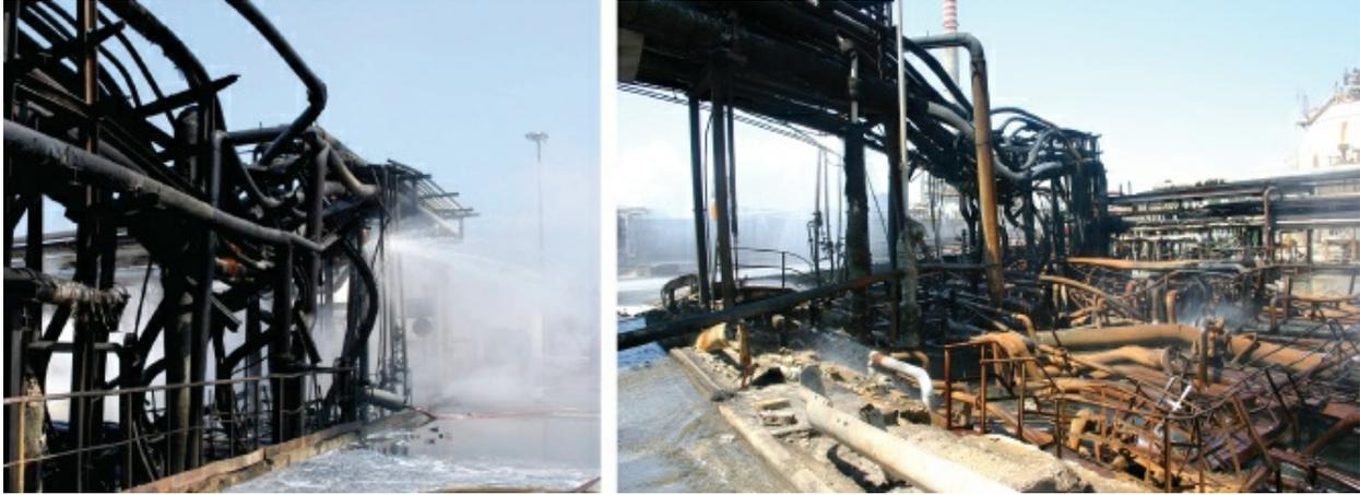
[Figure 7.4.2](#) Some damaged pipes downwards the road. There is also the pipe of the fire system.
