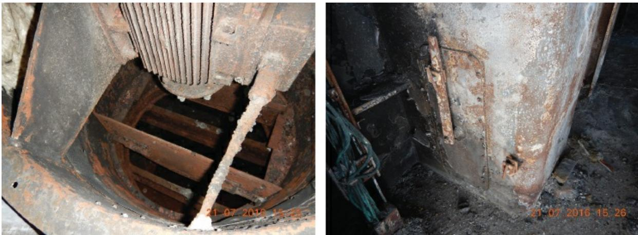
[Figure 7.2.2](#) Left: open fire damper of the garage ventilation. Right: local command at deck 4 for closing the fire dampers.
