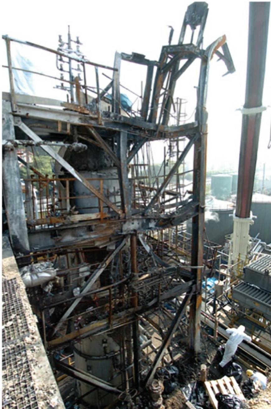
[Figure 7.8.4](#) Steel structure damaged
