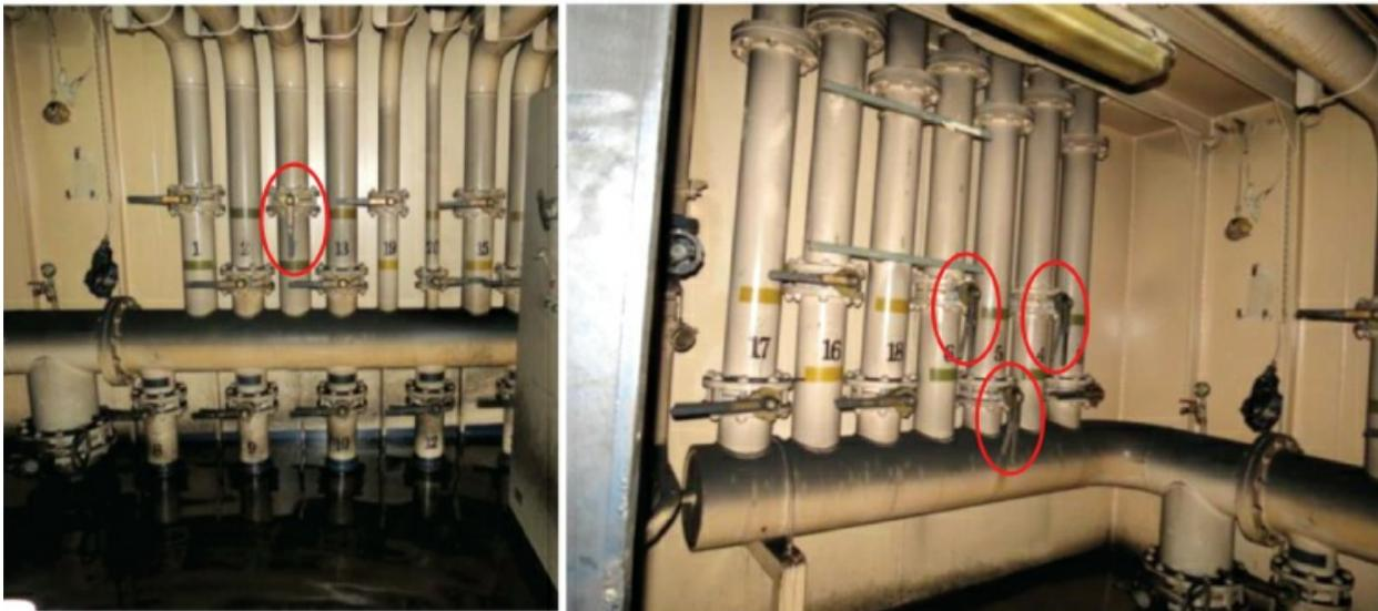
[Figure 7.2.4](#) The valves opened in the valve house are those activating the drencher at deck 3 (instead of deck 4).
