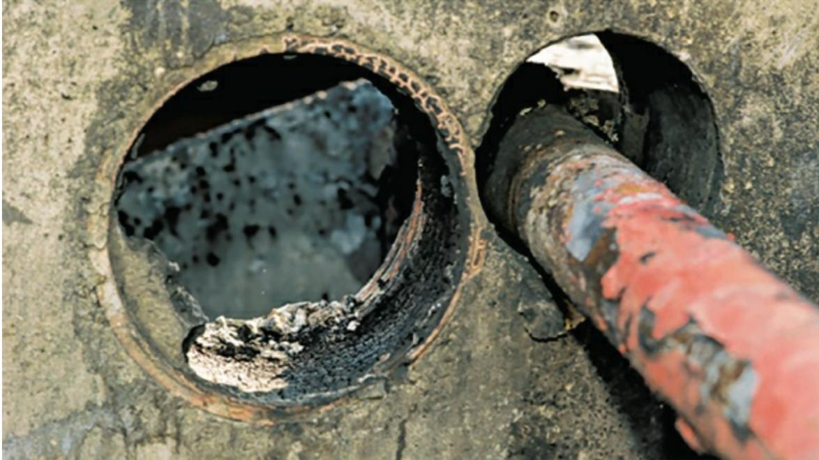
[Figure 2.44](#) Pipe penetrations for the loss of seal between pipes and walls.
