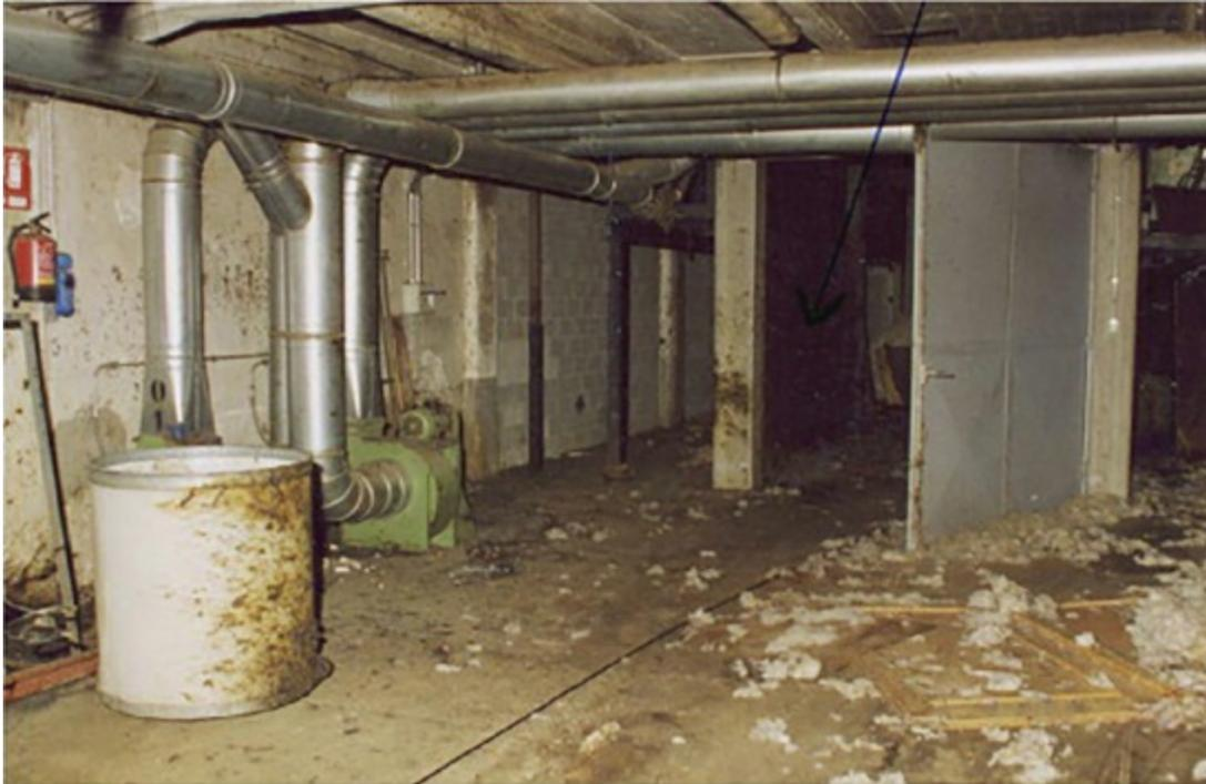
[Figure 4.23](#) Explosion of wool burrs, state of places, burrs collection boxes corridor with visible in the foreground signs of material fragment projection on the white bin.
