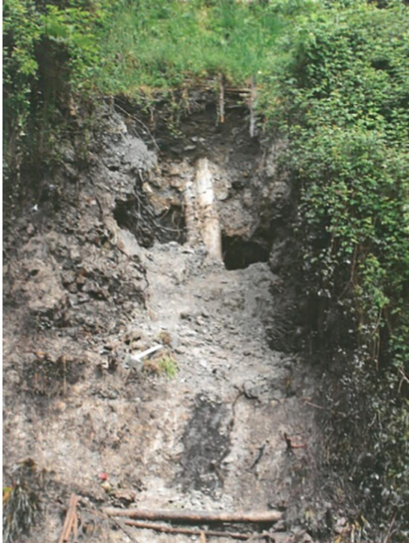
[Figure 7.9.1](#) Oil Pipeline near Genoa, affected by the rupture. It is evident the crater formed in the soil due to leaked oil pressure.
