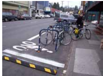
Portland is moving toward a simplified design with a single rubber curb, a pavement marking, and stripes to delineate the space. At each end, bicycle symbols with arrows direct traffic flow entering and exiting the corral. Photo: Greg Raisman
