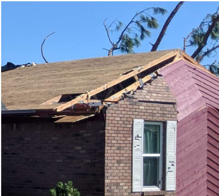
Gable-end Roof Damage
