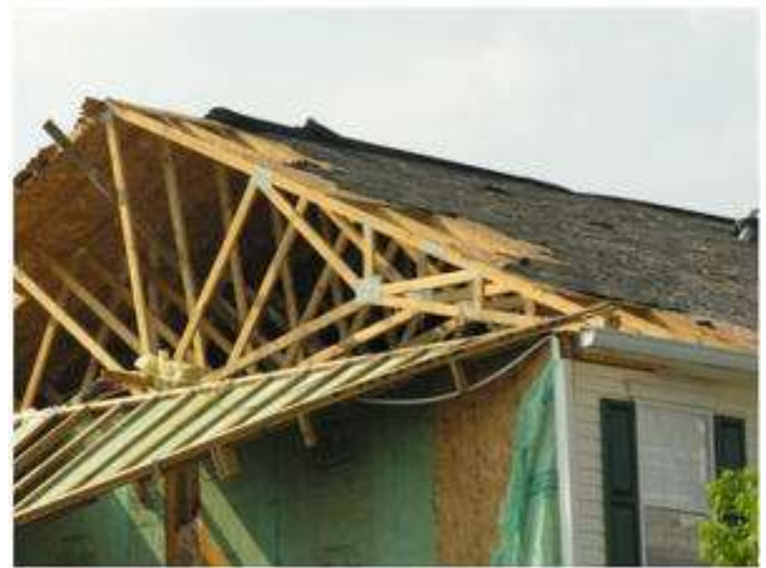
Gable-end Roof Damage
