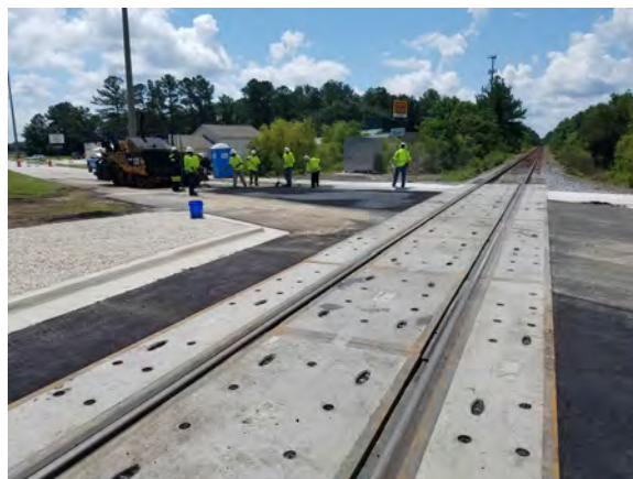
Overseeing CR 220 CSX Rail Replacement Project
