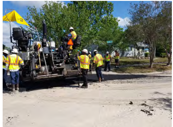
Repaving Project: Paving Doshire Drive
