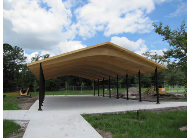
Construction of Pavilion at Moody Avenue ADA Park
