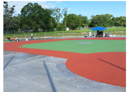
Installation of ADA Matting at Moody Avenue ADA Park
