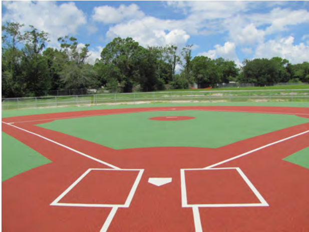
New Baseball Field at Moody Avenue ADA Park
