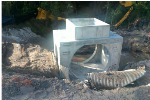
Inlet Installation for Pepperfish Drive Cross Drain Replacement
