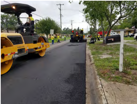
Repaving Project: Clermont Ave South
