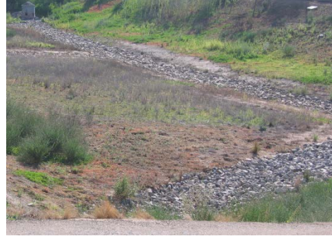
Figure 3: Gravel filled low-flow trench
