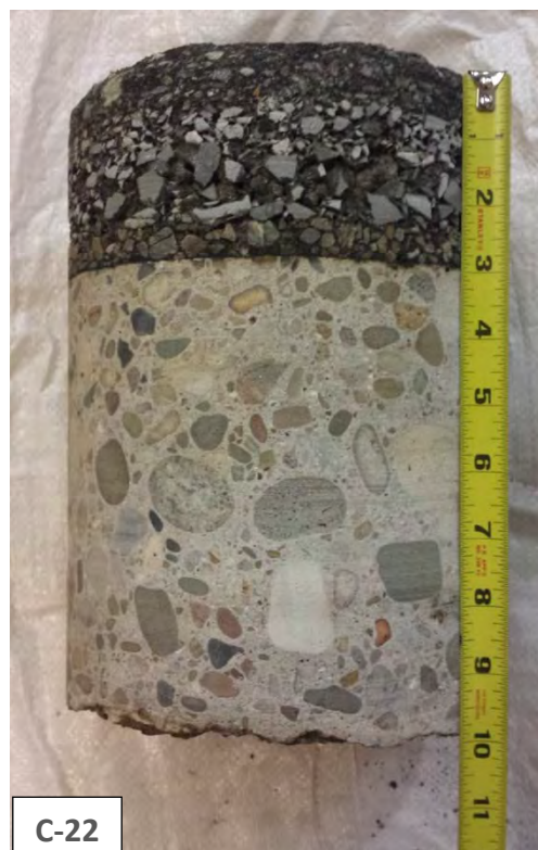
Figure 26-6 | Example of Pavement Core
