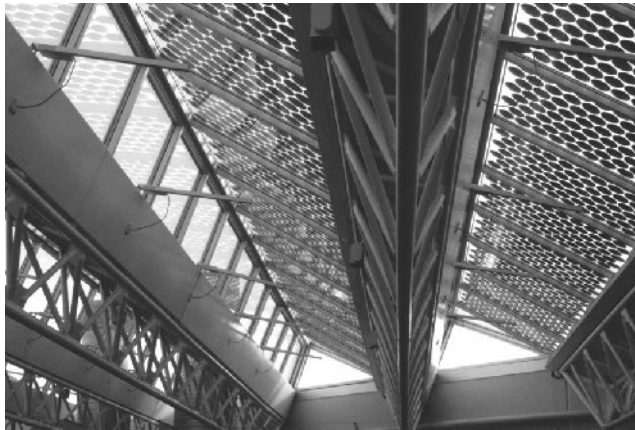
Figure 22.31 Atrium roof of the Brundtland Centre building from the inside. Because the saw-tooth roof casts a shadow on the modules, some of the cells are fake. This solution achieves a more elegant look from the inside. Reproduced with permission by BEAR Architekten T. Reijenga
