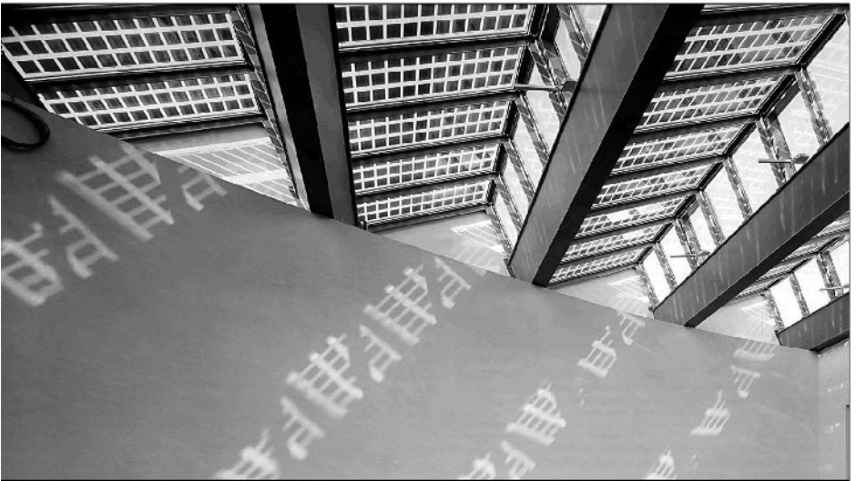
Figure 2.8 Photovoltaic integration into the glazing of a shed roof. In this case, photovoltaic cells serve also as optical shading elements for the space below, preventing overheating under summer conditions
