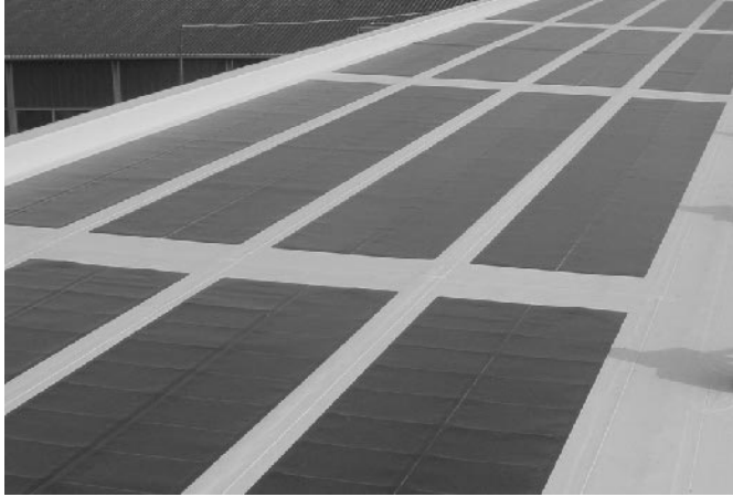
Figure 22.36 Alwitra Evalon® roofing foil with amorphous silicon cells. Reproduced with permission by O.Ö. Energiesparverband
