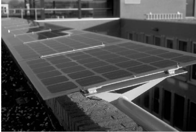
Figure 22.42 Canopy at the eaves of a roof. 6.2 kWp PV system at an office building in Gouda (NL). Reproduced with permission by BEAR Architecten T. Reijenga
