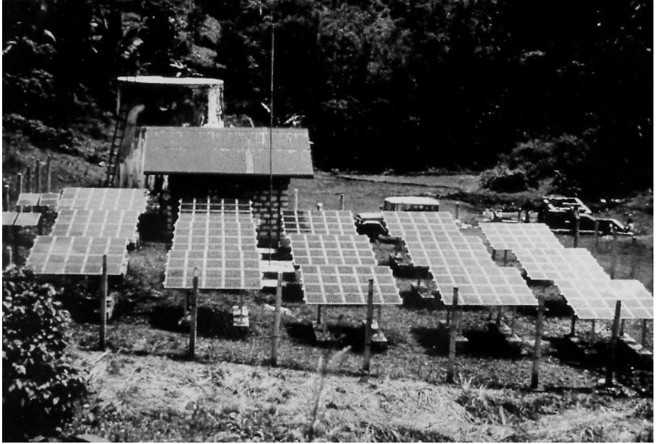
Figure 17.16 Photovoltaically powered system to provide drinking water for 4000 people (Source: TÜV Rheinland, Cologne)
