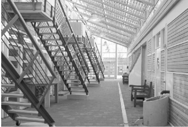
Figure 22.14 Corridor in the Centre for Sustainability De Kleine Aarde in Boxtel (NL). The space is unheated and naturally ventilated. The 6.7 kWp PV system with transparent modules has a double function and reduces the heat load by around 70%. Reproduced from Reijenga T, Böttger W, Proc. 2 nd WC Photovoltaic Solar Energy Conversion , 2748–2751 (1998) with permission by NOVEM, R Schropp [11]
