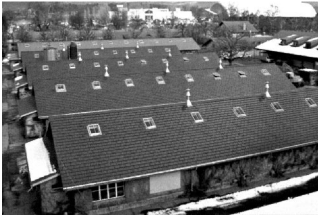
Figure 22.15 The 80.5 kWp Atlantis Sunslates on the roof of the historic horse stables in Bern (CH). The color and texture matches so well that this PV system was allowed on a protected historic building. Reproduced with permission by Atlantis Solar Systems Ltd
