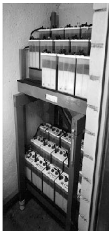
Figure 18.11 A battery in a photovoltaic system with a rated capacity of C_{10} = 37.5 Ah and a rated voltage of 168 V (flat-plate technology, 28 blocks of 6 V connected in series, Picture courtesy Fraunhofer ISE)
