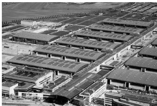
Figure 17.28 Central PV system installed on the roof of the new fair in Munich, Germany (Source: Siemens Solar)
