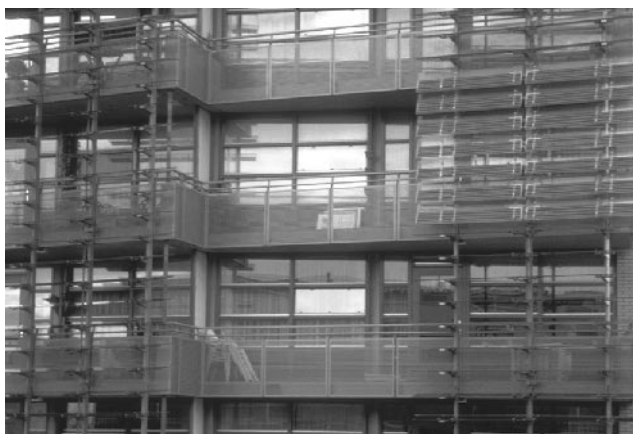
Figure 22.41 ADO louver system with integrated transparent PV modules at an apartment building in Amersfoort Nieuwland (NL). The automatic louvers can switch in two positions. The horizontal position at night (left on the figure) and tilted to the sun by day (right on the figure). Reproduced with permission by BEAR Architecten T. Reijenga
