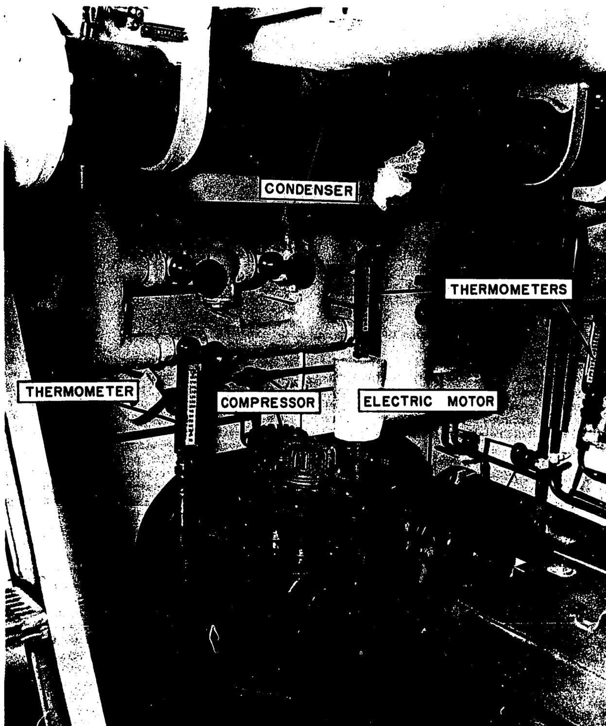
Figure 19-3.—High pressure side of R-12 installation aboard ship.
