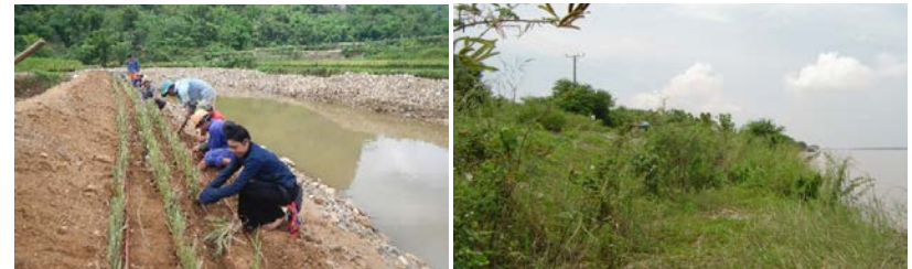
Riverbank stabilization. Vetiver grass planted along a riverside in northern Viet Nam (left) and the grassed flood foreshore with small trees on an embankment in Cambodia (right) provide for riverbank stabilization (photos by the International Centre for Environmental Management and J. Howell).
