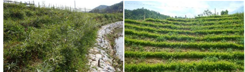
Strongly rooted plants. In northern Viet Nam, the method adopted of propagating shrubs and small trees for shallow stabilization of unconsolidated slopes is one that makes the plants produce a mass of fine, strong roots, which provide soil reinforcement. (photos by the International Centre for Environmental Management).
