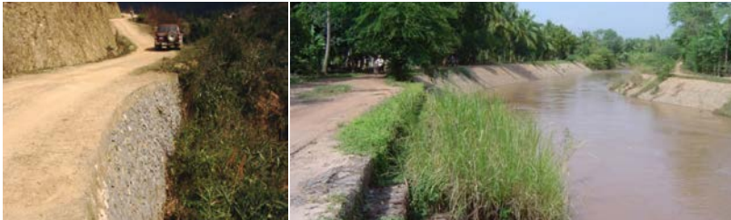
Grass slope protection. In Viet Nam, large grasses are planted to prevent erosion below the toe of a road retaining wall. In Cambodia (right), grass planted on the bend of an irrigation canal is among the different methods of bank stabilization (photos by J. Howell).
